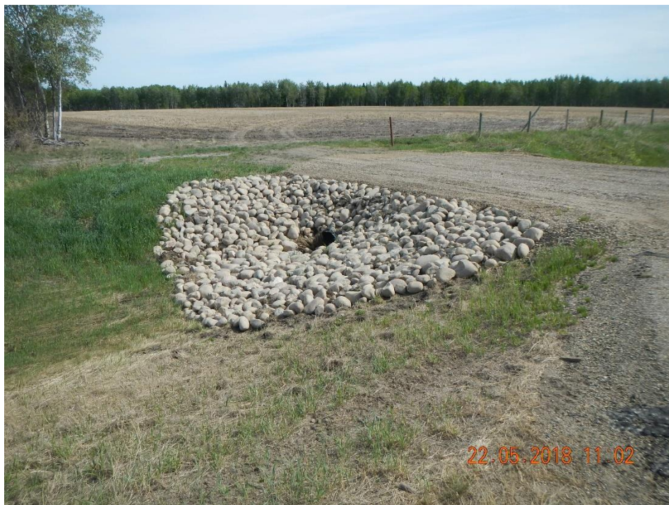
Photo 4 (MCI, May 22, 2018) – Looking northeast at restored approach and culvert inlet riprap.
