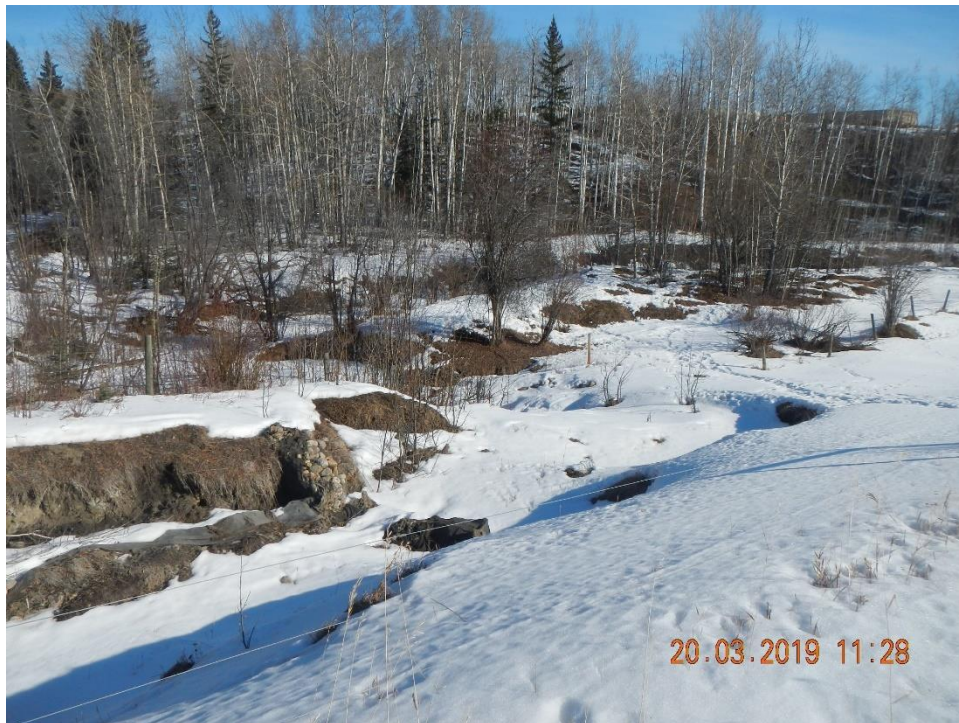
Photo 8 (MCI, March 20, 2019) – Looking north at remnants of the erosion protection.
