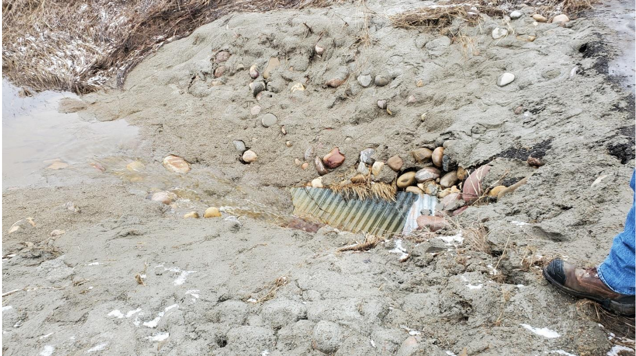
Photo 11 (April 28, 2022) – Grouted riprap at the approach culvert inlet.
