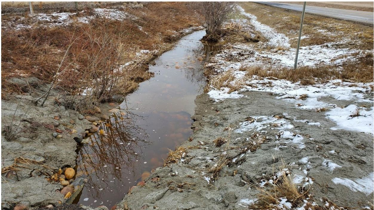
Photo 12 (April 28, 2022) – Looking downstream (east) from approach culvert outlet (riprap also grouted).
