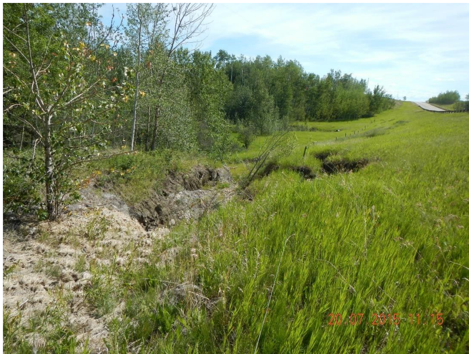
Photo 2 (MCI, July 20, 2015) – Looking east at erosion gully.
