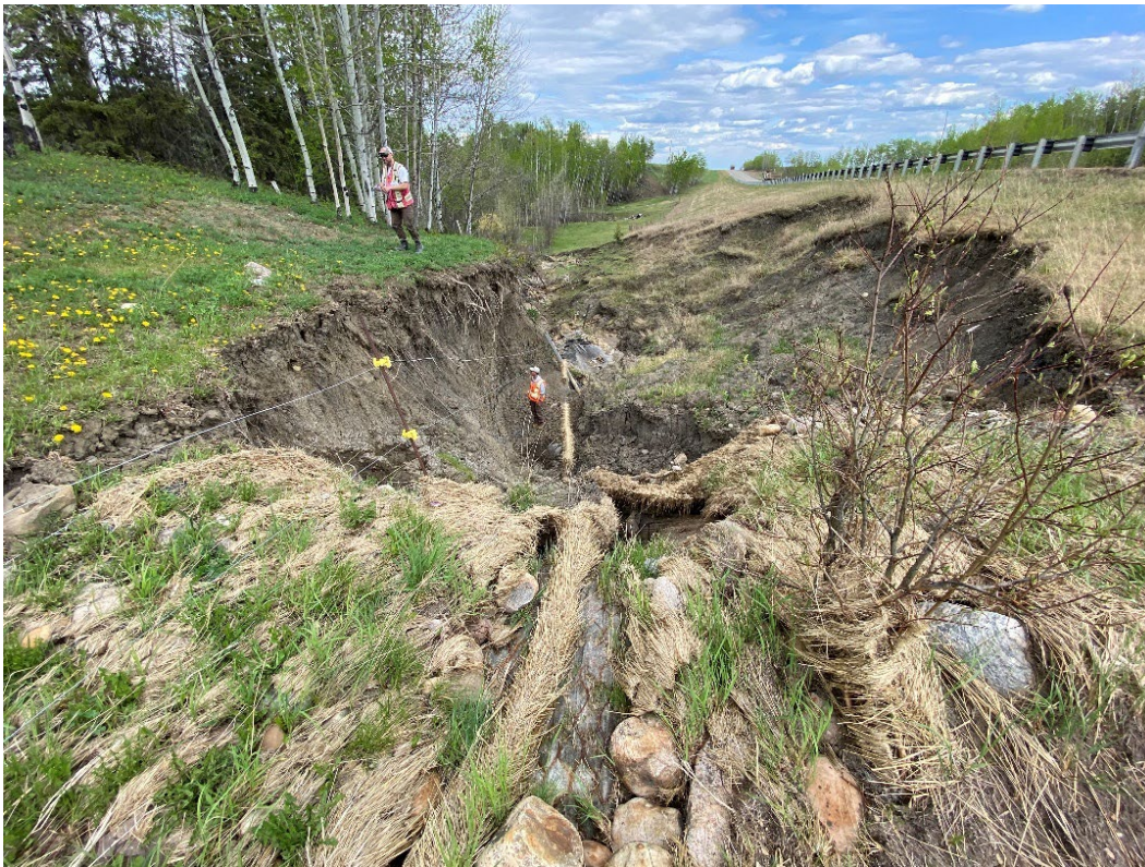
Photo 4 – Looking east along the north ditch and north hwy embankment at the beginning of the erosion where erosion gully slumping is closest to the highway.
