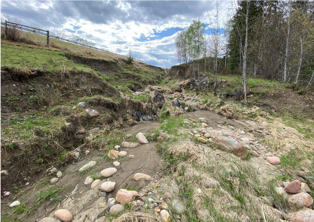
Photo 5 – Looking southwest at the runoff erosion gully in the north hwy embankment, where the damaged gabion mattress and underlying nonwoven geotextile is exposed.
