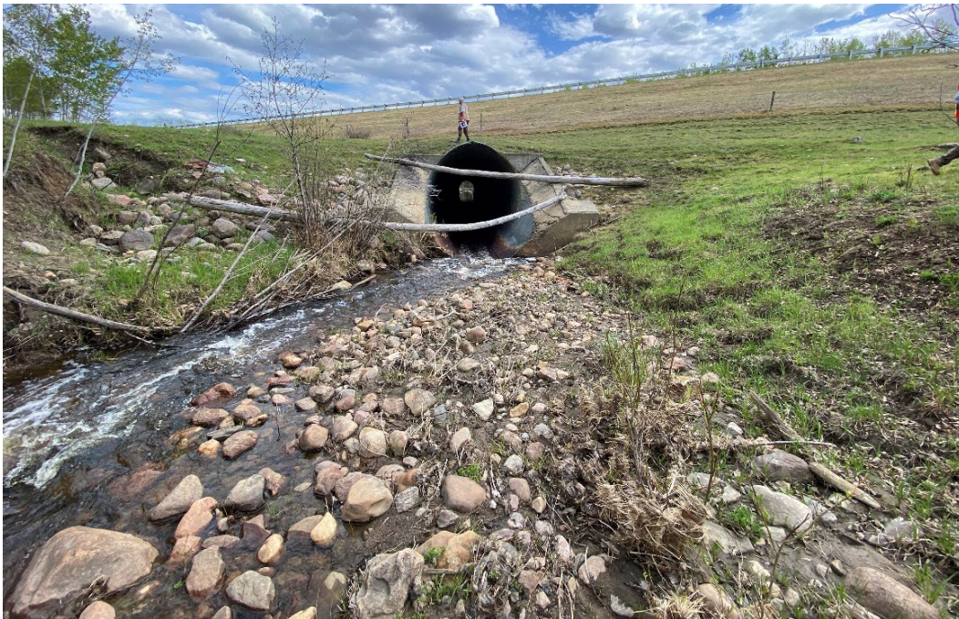
Photo 9 – Looking southeast at the inlet of the 3.5 m dia. BF culvert. Note the erosion gully on the east channel bank north of the entrance.
