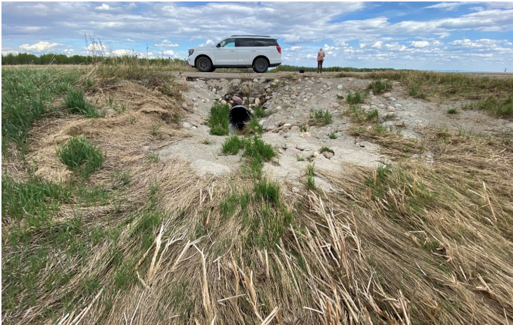
Photo 1 – Looking east at the grouted riprap at the inlet of the 800 mm dia. culvert at km 2.845 approach.
