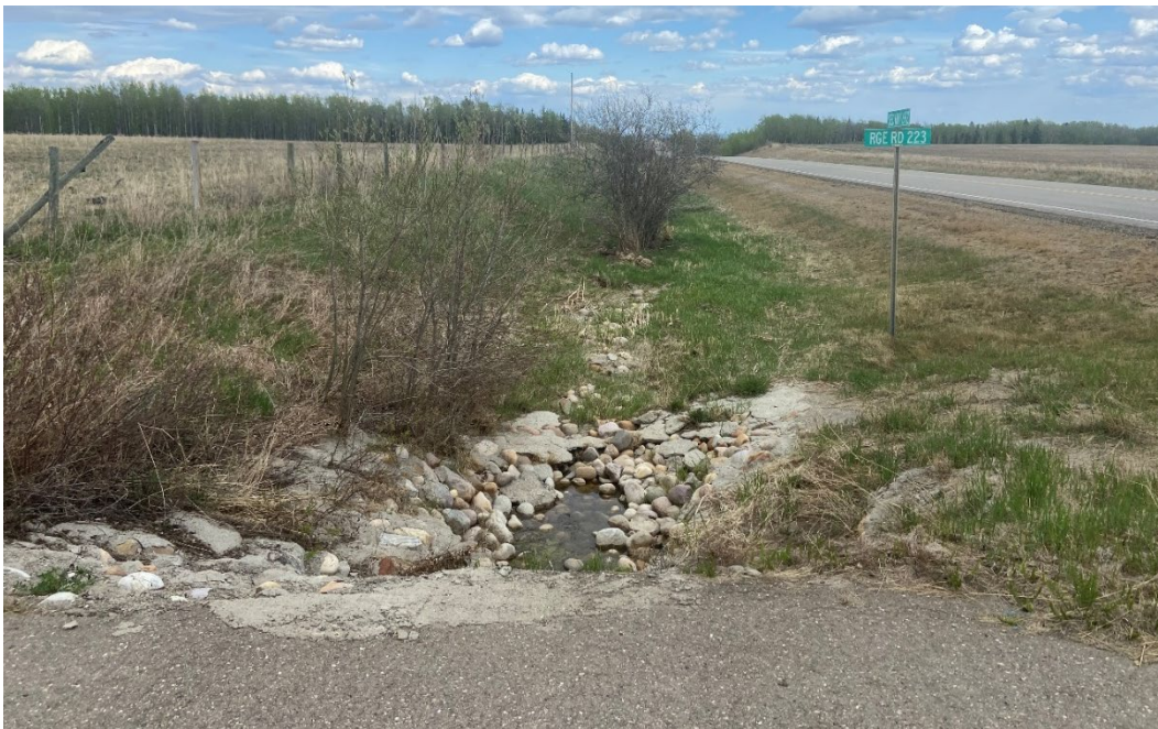
Photo 2 – Looking east along the north ditch over the outlet of the culvert at the km 2.845 approach. Note the standing water.
