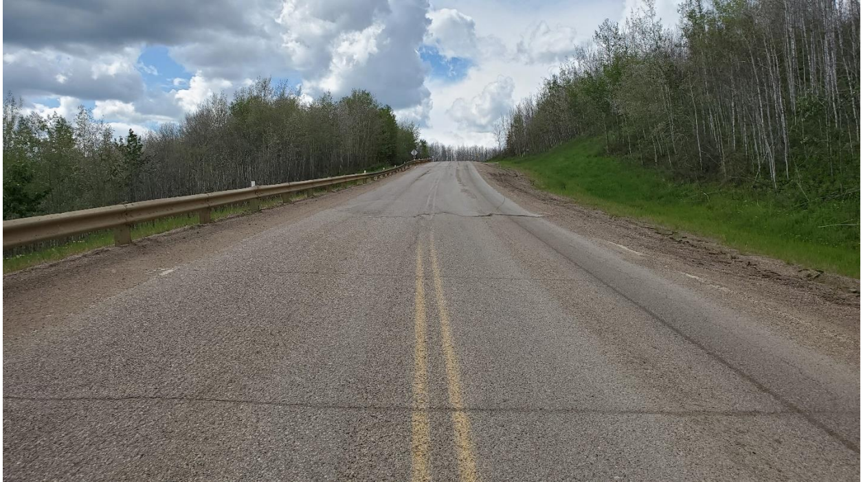
Photo 5 – Looking southwest at recent patch near southwest portion of the site.
