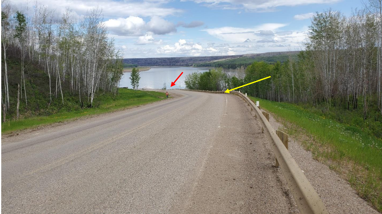
Photo 7 – Looking east at dips in the road (minor with yellow arrow, major with red arrow).
