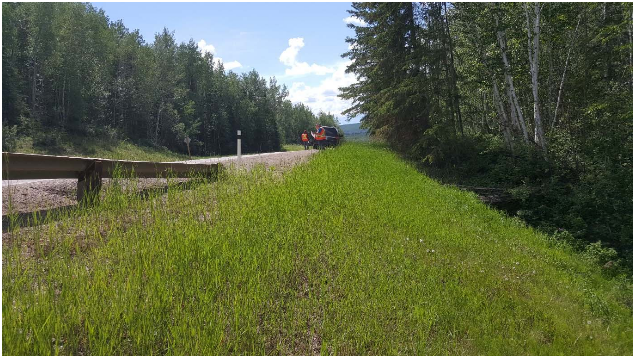
Photo 4 – Looking southwest at northwest sideslope.
