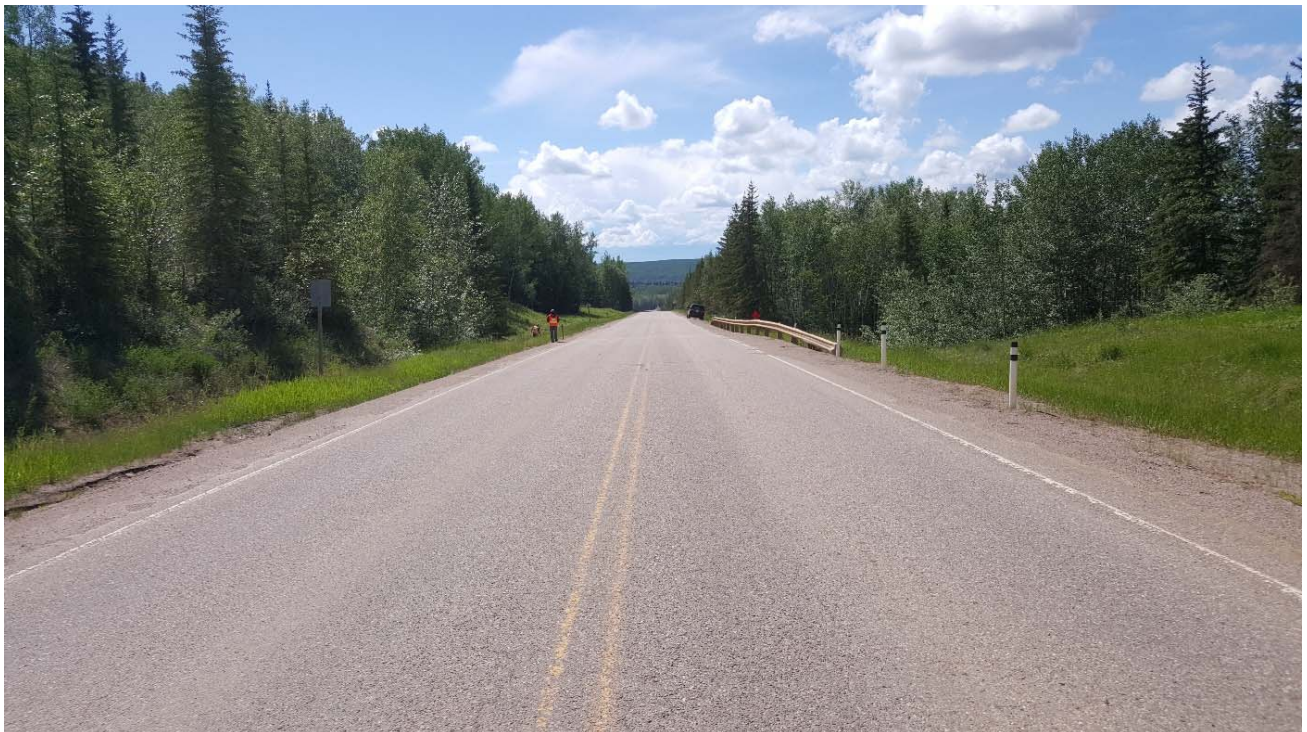
Photo 2 – Looking southwest from northeast end at dip in highway.
