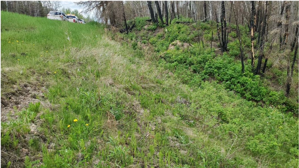
Photo 4 – Looking southwest at northwest sideslope.
