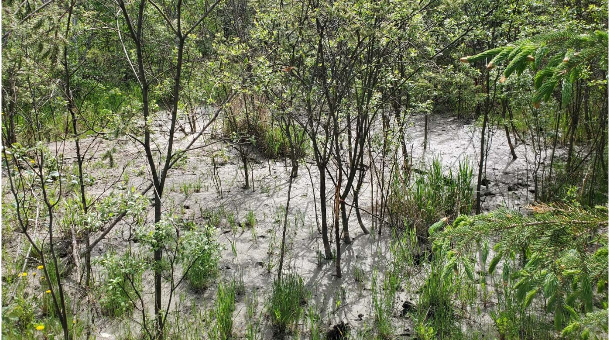
Photo 5 – Silt accumulation upslope of inlet.
