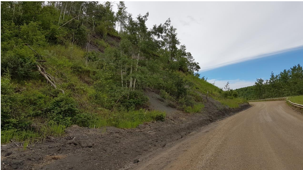
Photo 8 – Looking southeast at ravelling shale slope (km 43.2).
