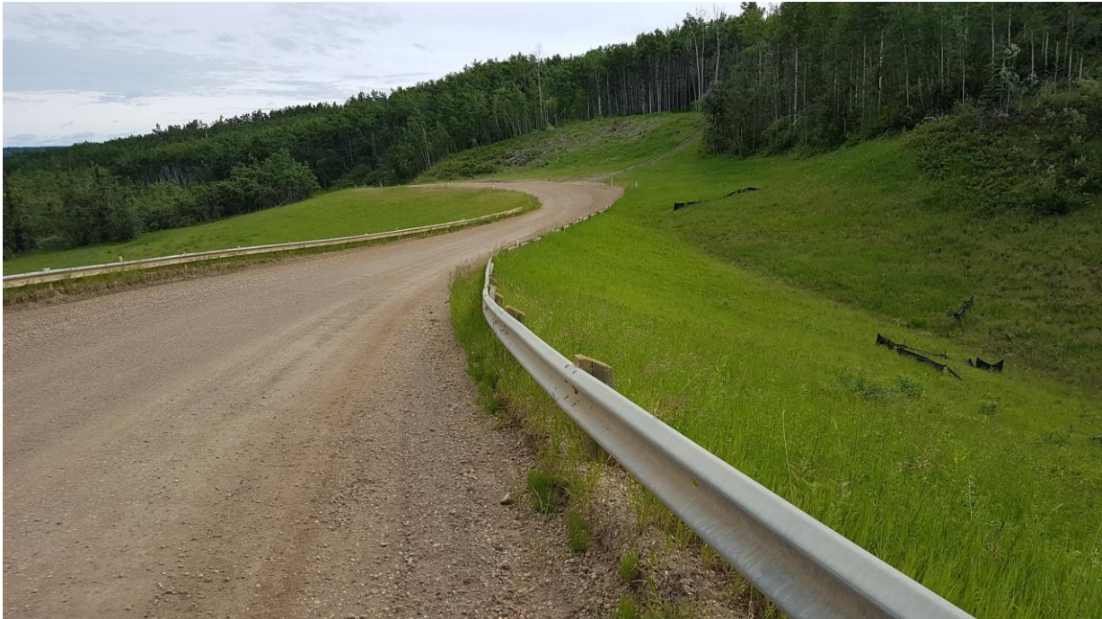
Photo 5 – Looking north at along east guardrail.
