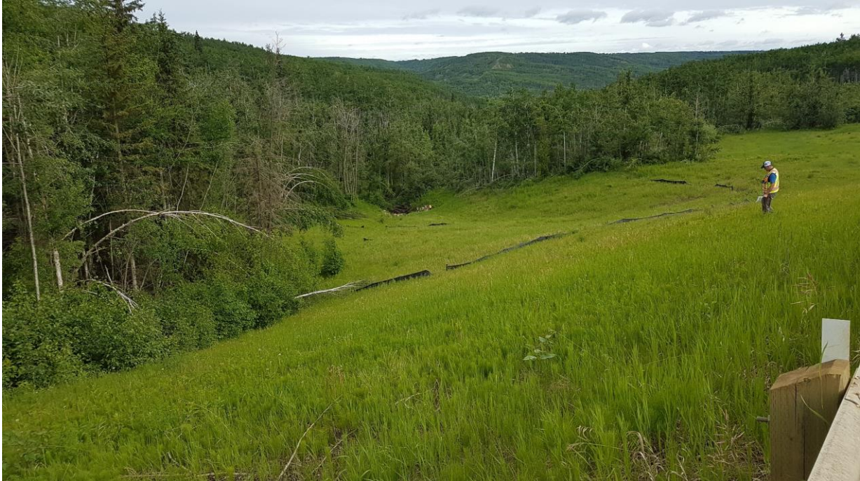
Photo 3 – Looking west toward culvert outlet along west sideslope.
