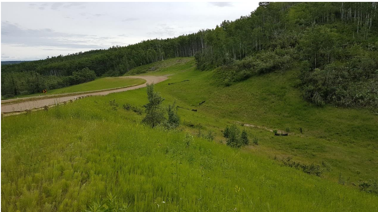
Photo 4 – Looking north at east sideslope above culvert inlet.
