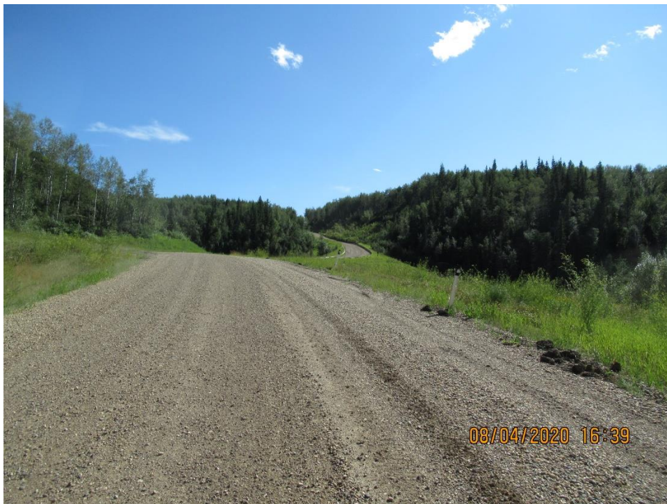
Photo 6 – Looking south at hump in road profile south of the site.
