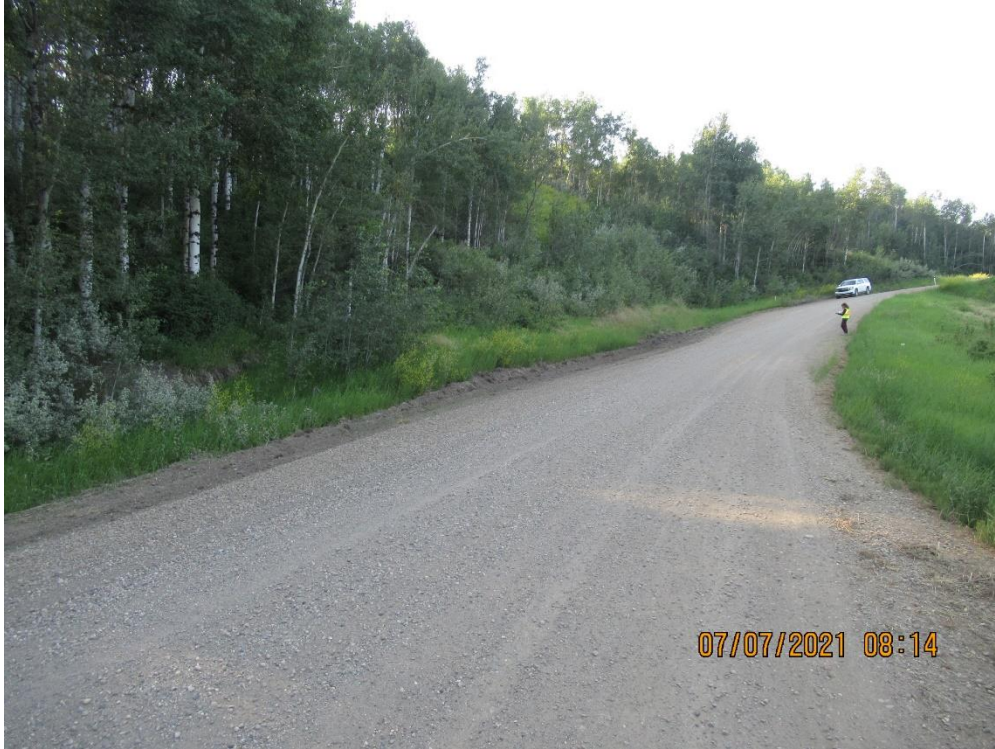
Photo 5 – Looking south toward the landslide.
