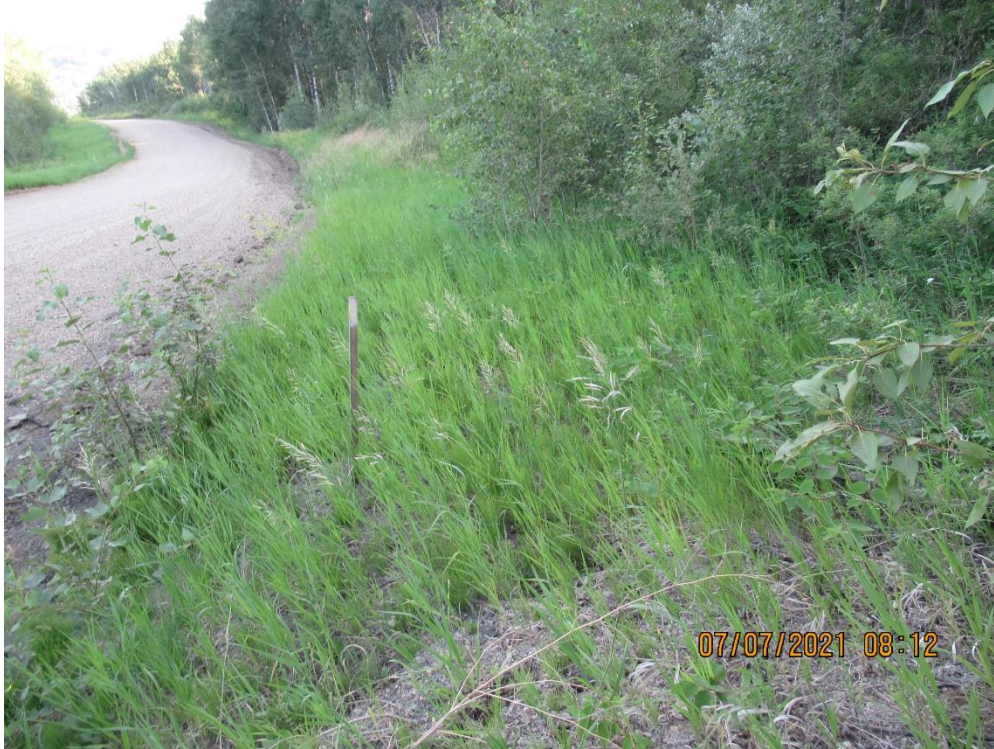
Photo 3 – Looking north along backscarp crack (in the grass).
