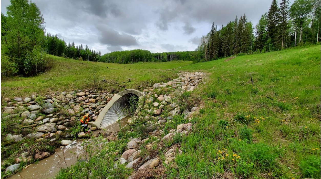
Photo 3 – Looking west at culvert outlet.
