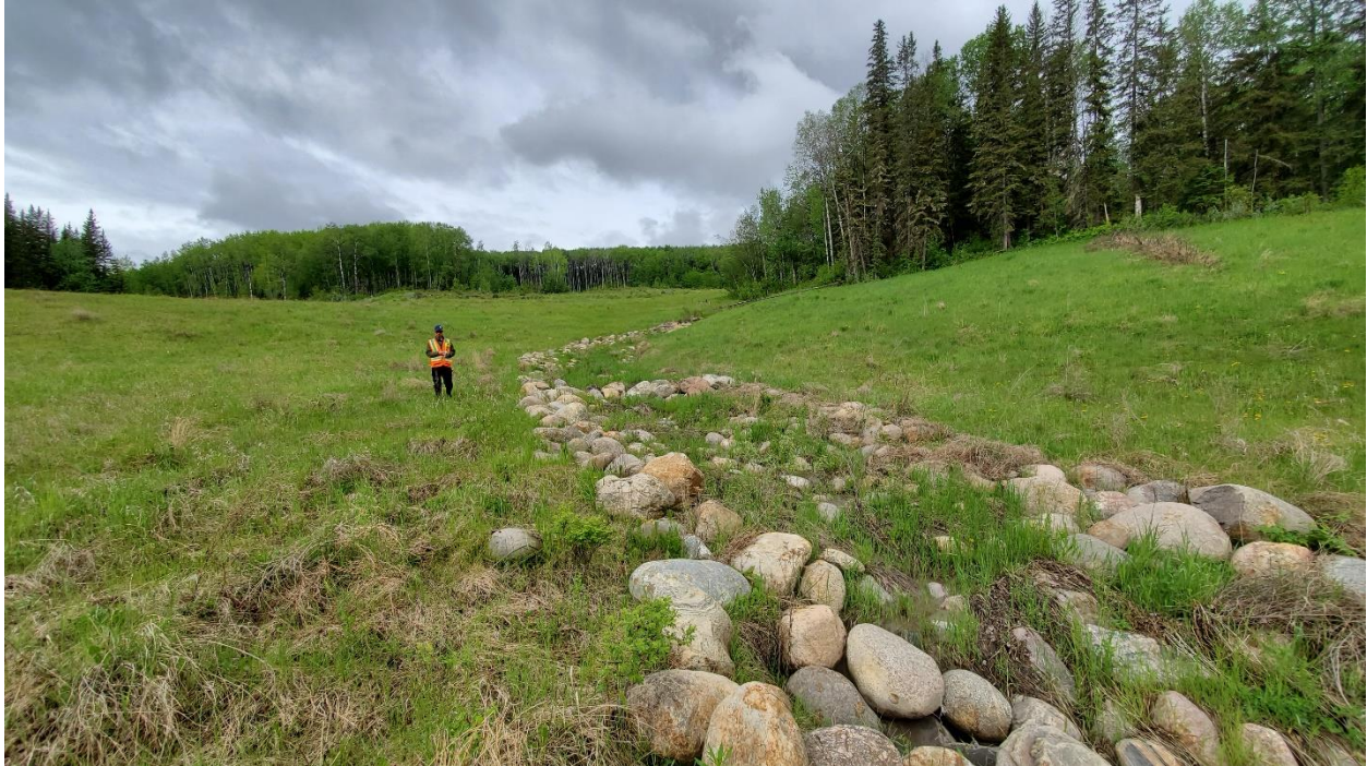
Photo 5 – Looking west at swale near the culvert outlet.
