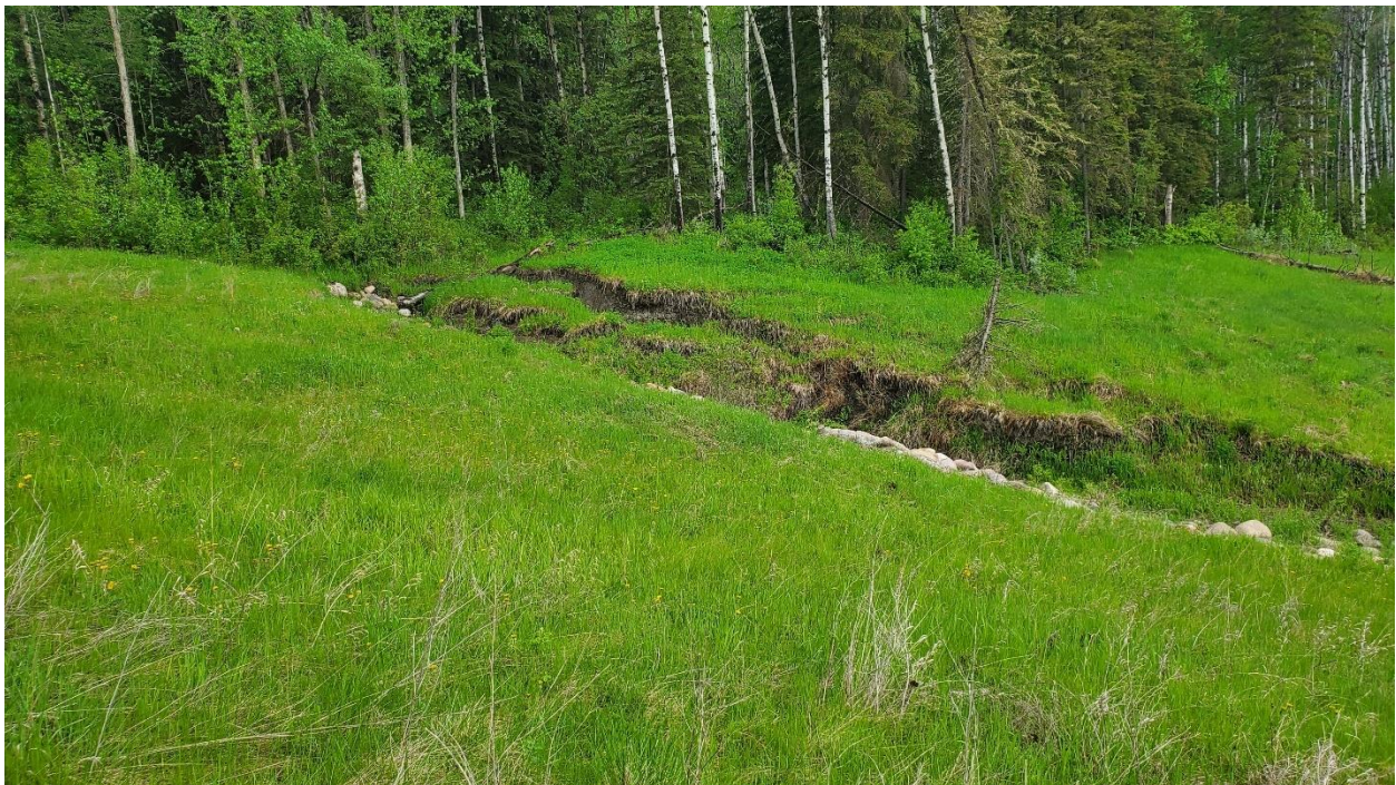
Photo 2 – Looking north at erosion on north side of drainage swale.
