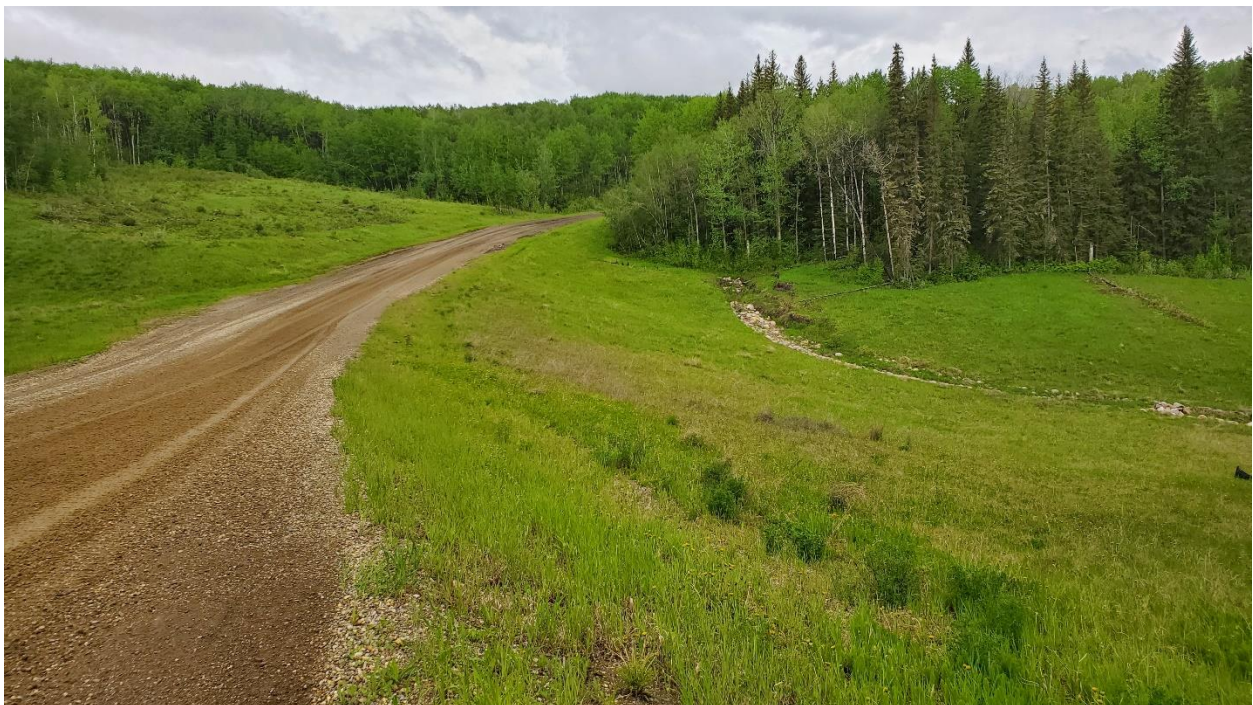
Photo 6 – Looking northwest at road and north side slope.
