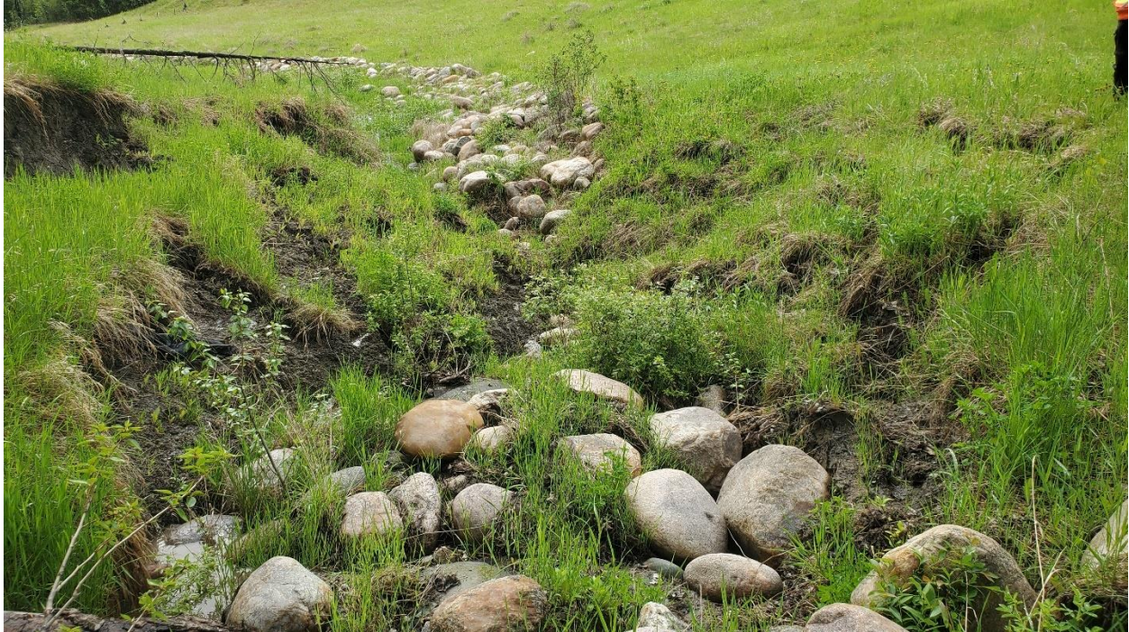
Photo 1 – Looking at west end of drainage swale.
