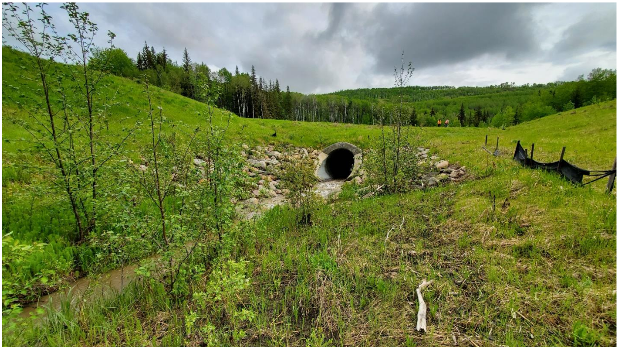
Photo 4 – Looking northeast at culvert inlet.
