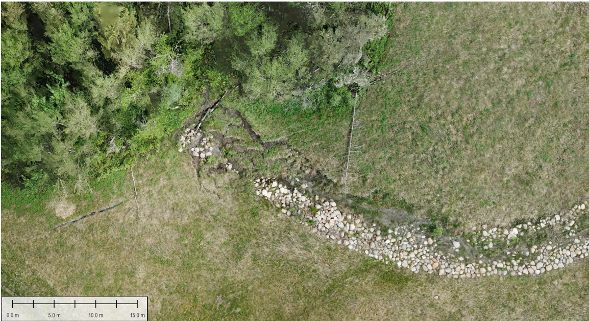
UAV 2020 Orthoimage – Slumping at start of riprap channel
