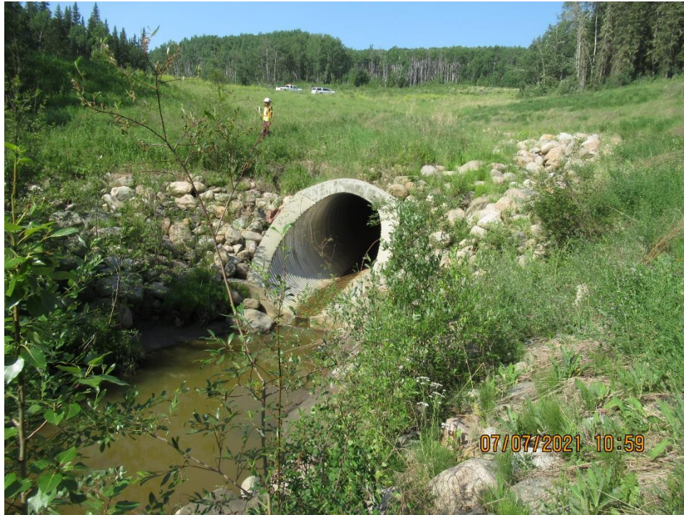
Photo 3 – Looking west at culvert outlet.
