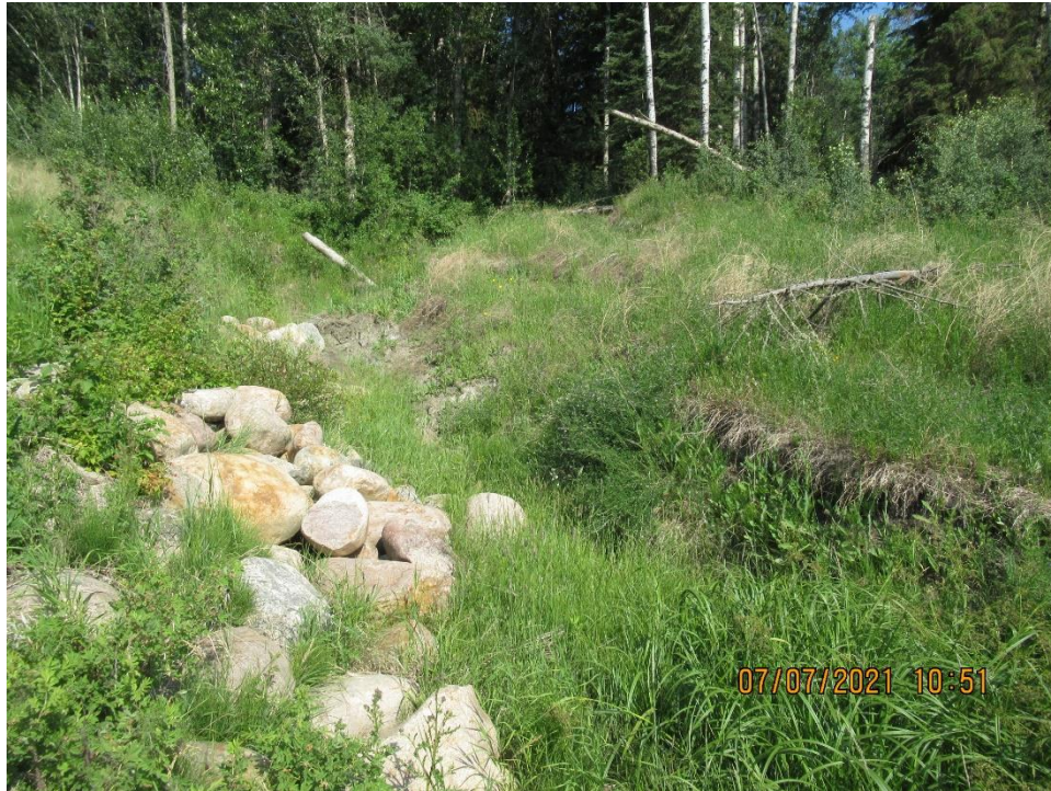
Photo 1 – Looking at west end of drainage swale.
