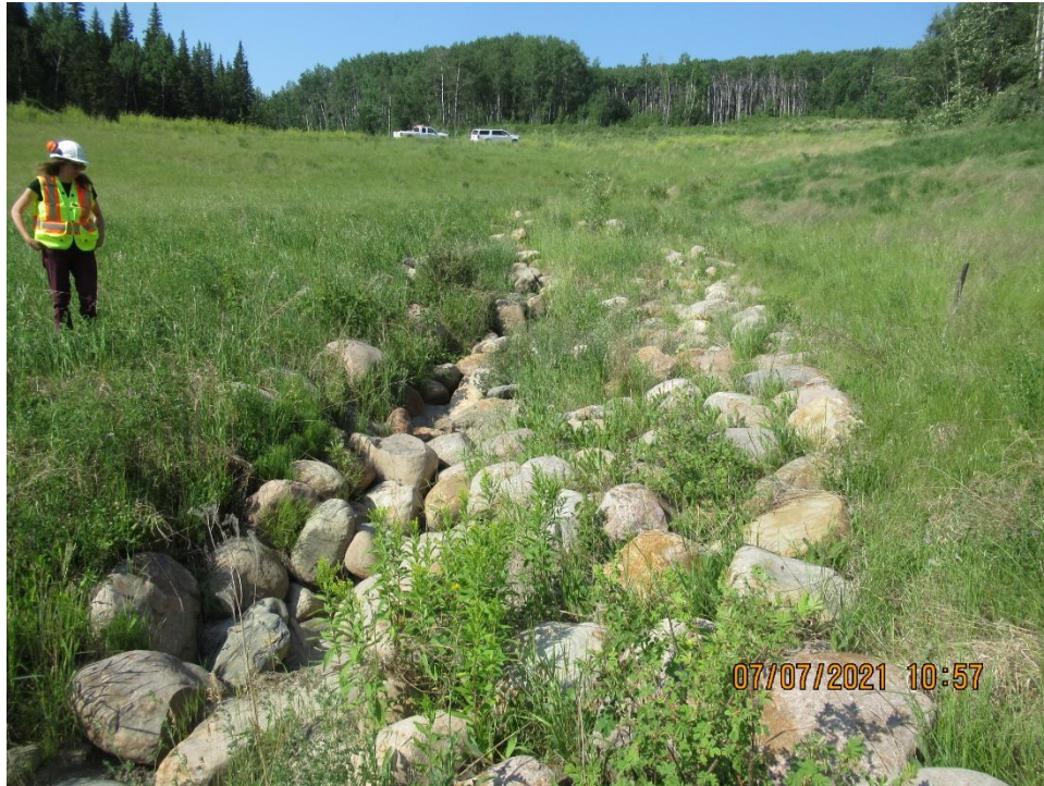
Photo 5 – Looking west at swale near the culvert outlet.
