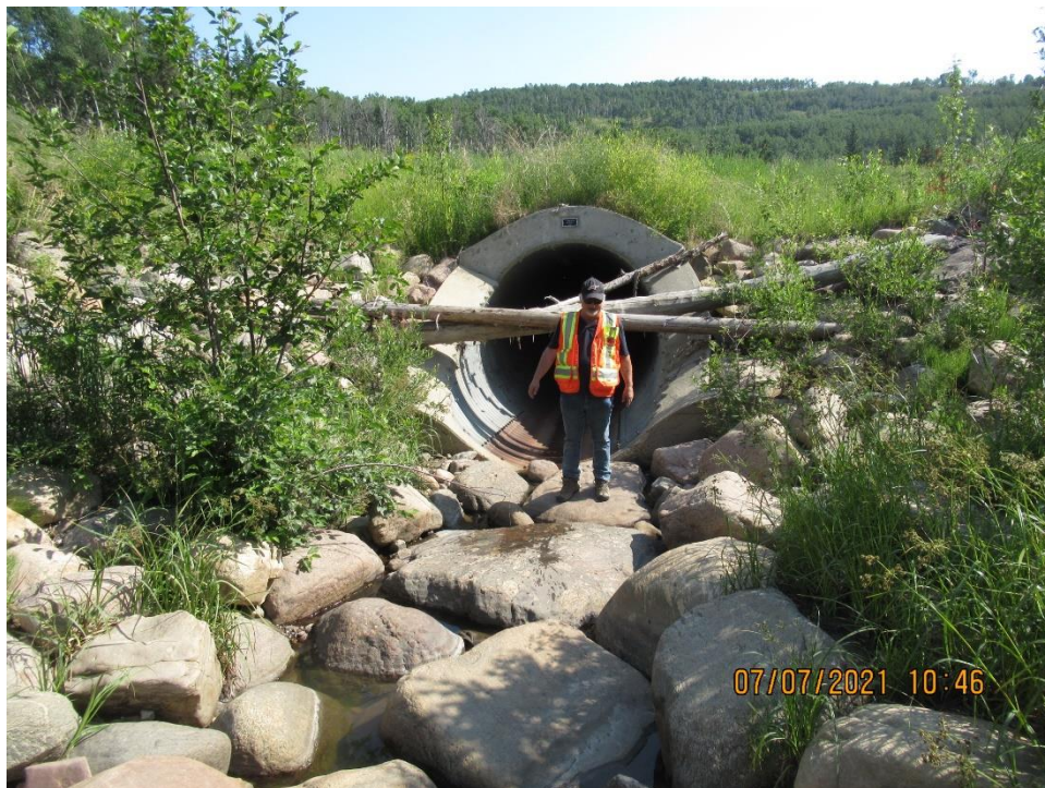
Photo 4 – Looking northeast at culvert inlet.
