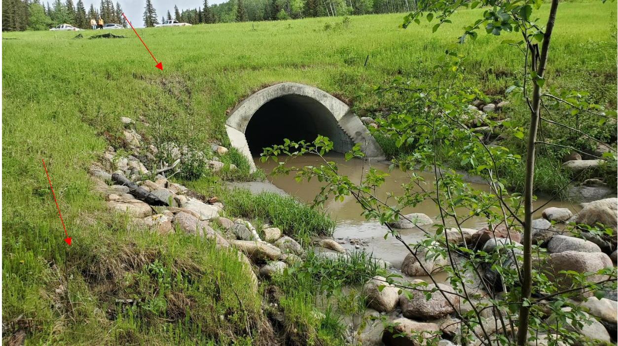
Photo 5 – Looking north at culvert outlet and shallow gullies (arrows)
