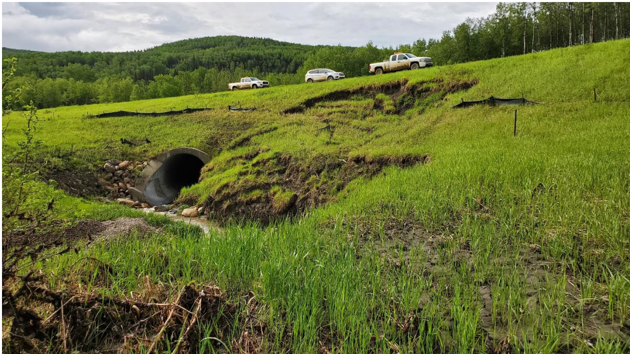
Photo 4 – Looking south at culvert inlet.
