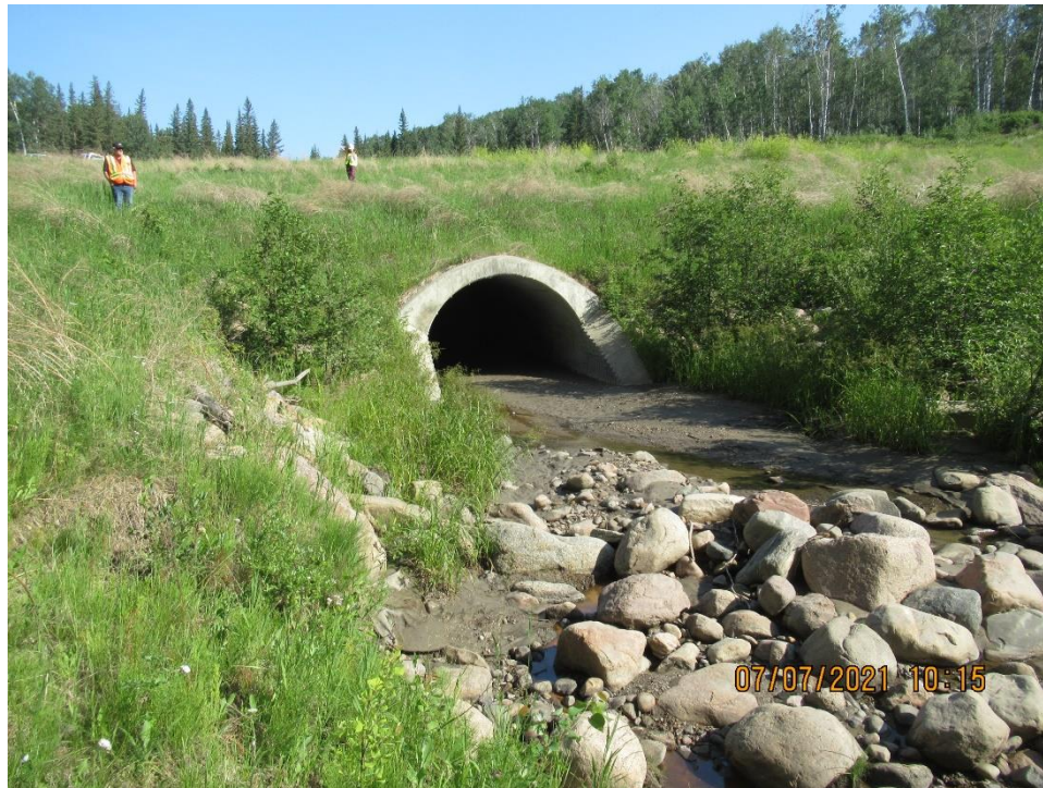
Site 1, Photo 5 – Looking north at culvert outlet
