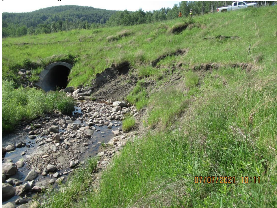
Site 1, Photo 4 – Looking south at culvert inlet.
