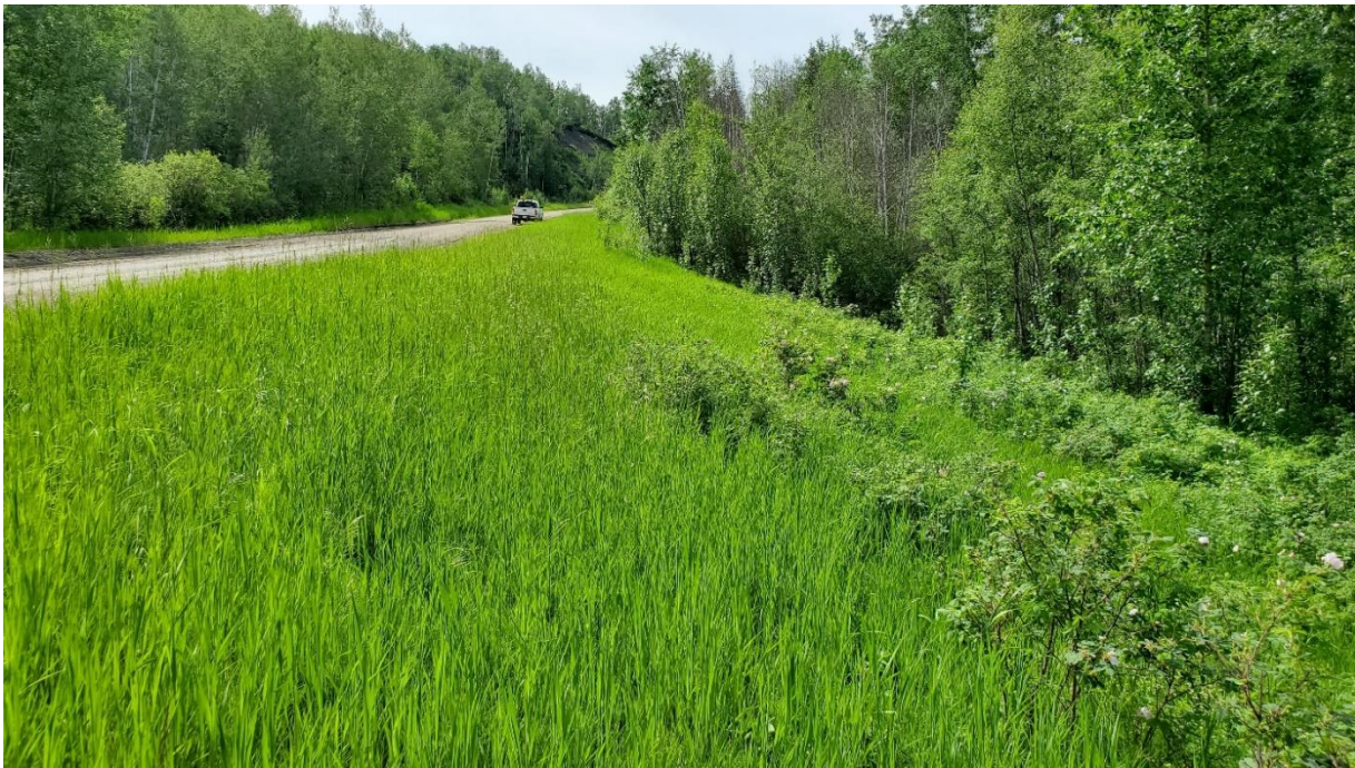
Photo 4 – Looking south at the sideslope of the highway below the slide.
