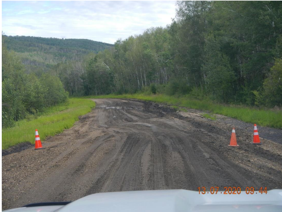
Kurz, July 13, 2020 – Looking south at PH087 site.
