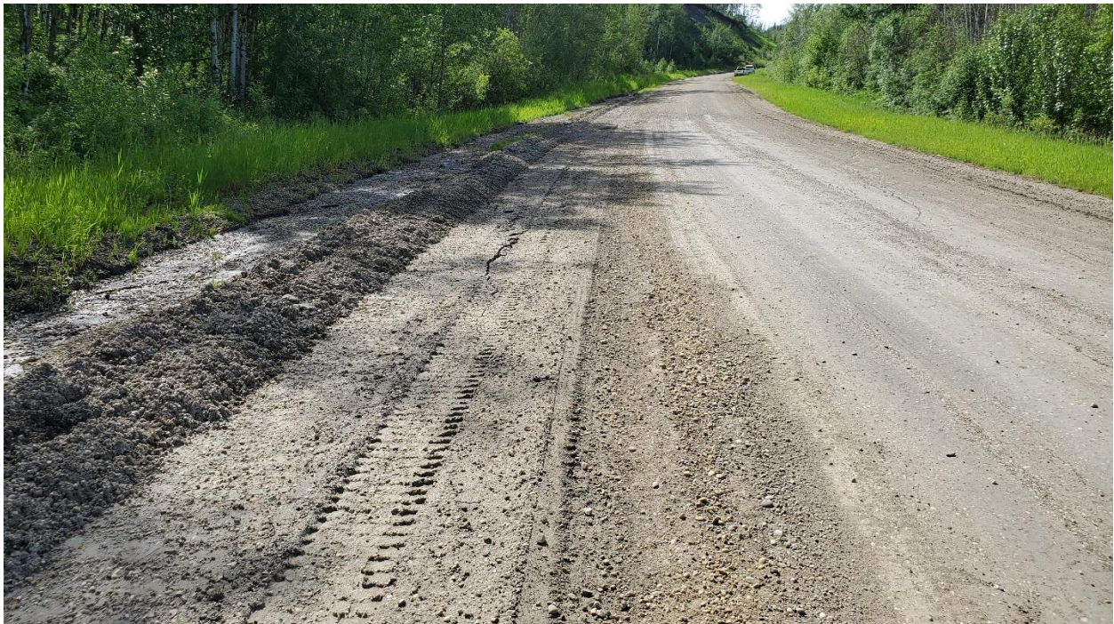
Photo 6 – Looking south at the main scarp crack in the east ditch. The "shale slope" sub-site of PH011 is visible in the background at the curve in the road.
