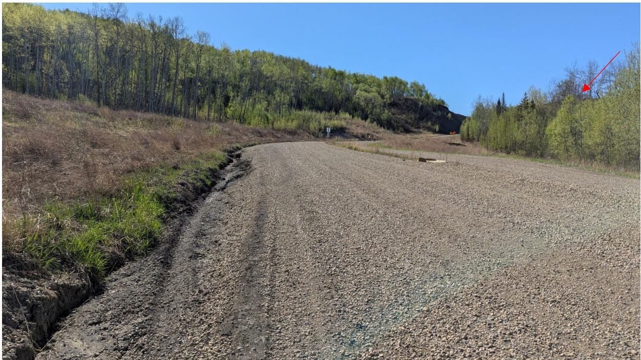
Photo 2 – Looking south along the alignment. Scarp through the old road denoted by arrow. Note that there is only a shallow v-ditch that has been cut by the grader and it is starting to downcut from erosion.
