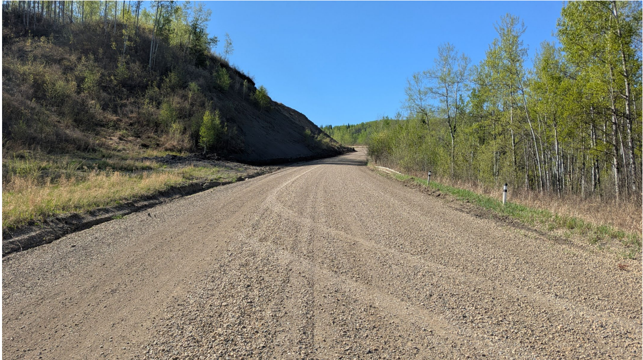
Photo 7 – Looking south towards the south landslide lobe and high shale backslope (PH011-2) on left. Ongoing grading has obscured the cracks at the guardrail from the south lobe of the slide.
