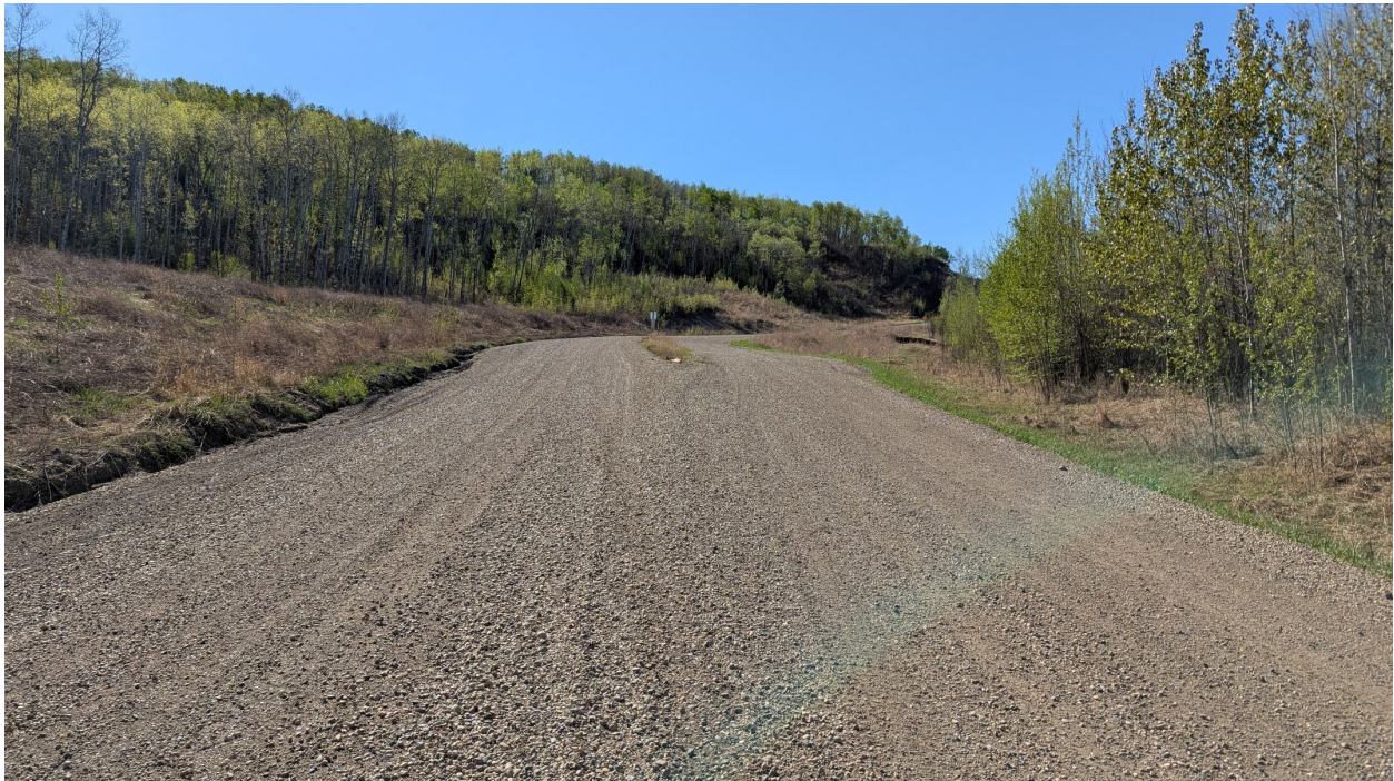
Photo 4 – Looking south at the north end of the detour where it splits around a previously-soft area. Upslope ditch has less erosion than at the previous inspection.
