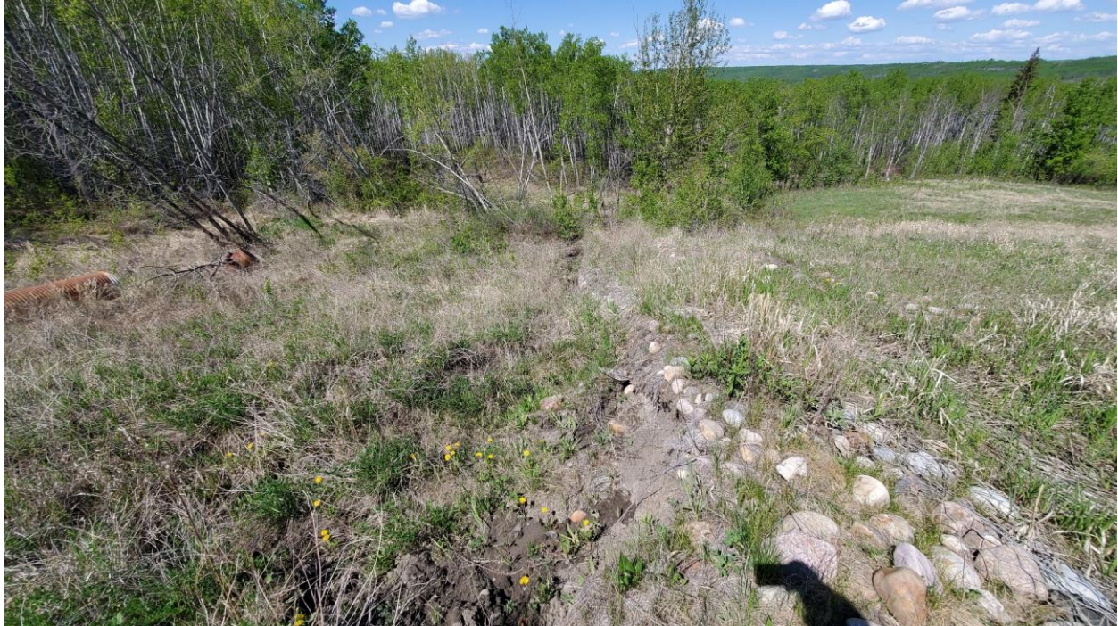
Photo 5 – Looking west where slide at km 14.45 cuts into the gabion basket swale.
