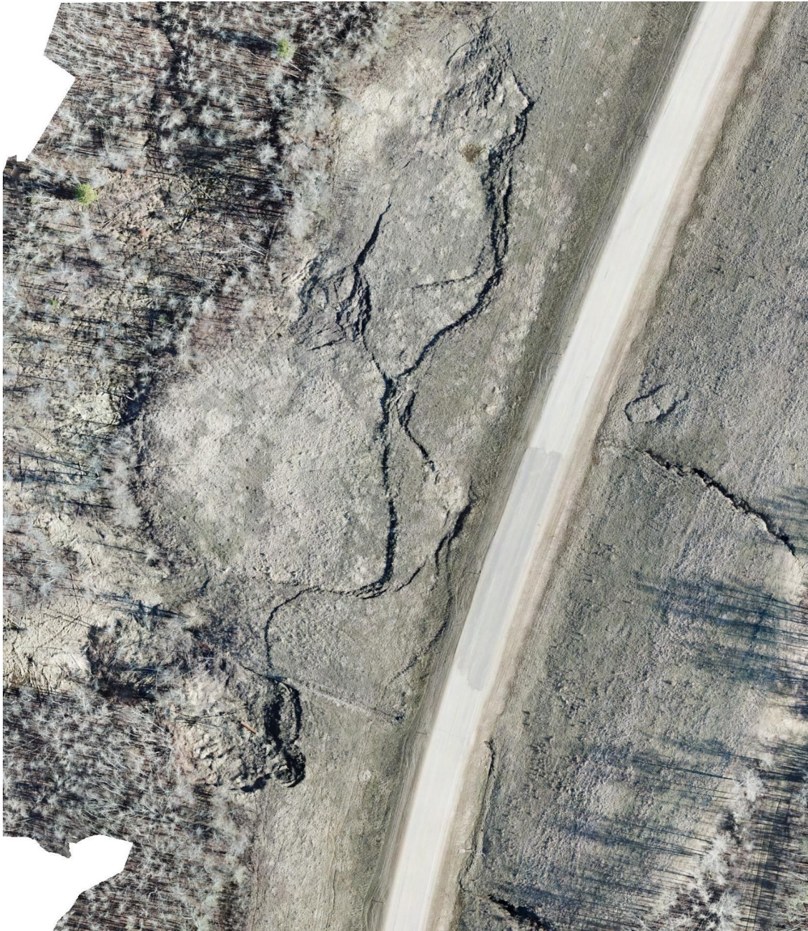
2022 UAV orthomosaic showing the developing landslides that have damaged the south gabion basket swale and are encroaching towards the highway.
