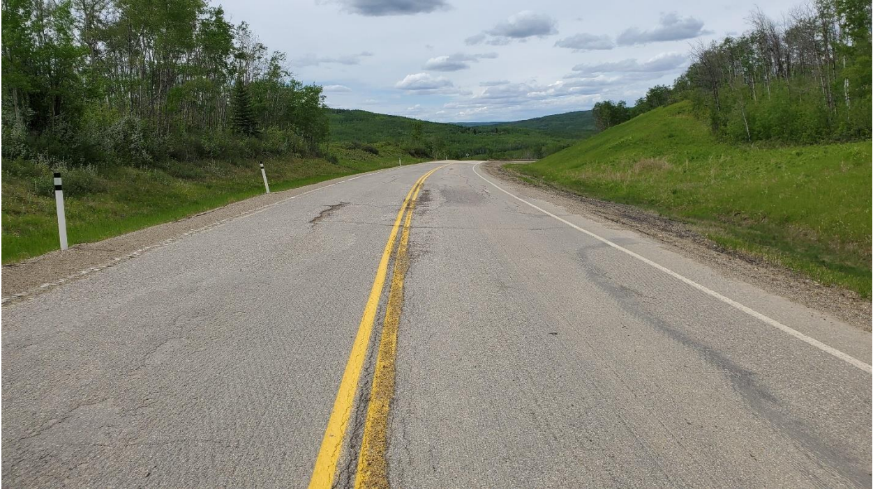
Photo 5, Site 4 – Looking west at patch at ~km 18.750.
