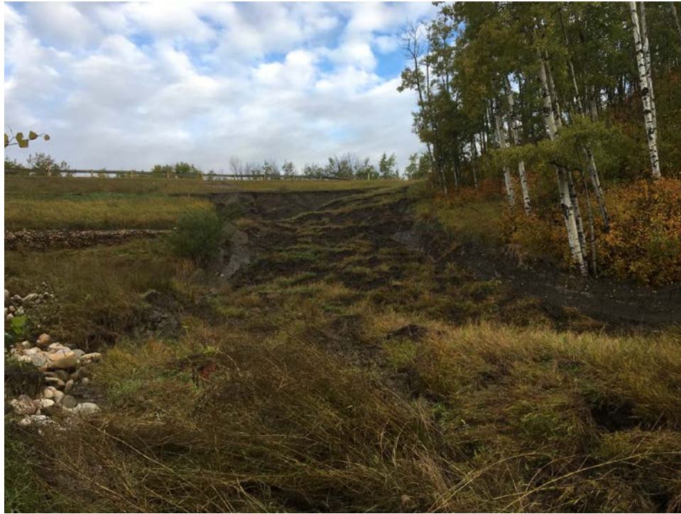
Photo 3: Looking northwest up at slide mass.
