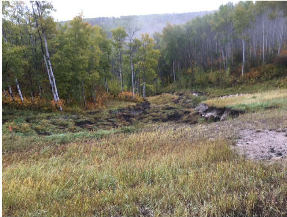
Photo 1: Looking east from the edge of the highway.
