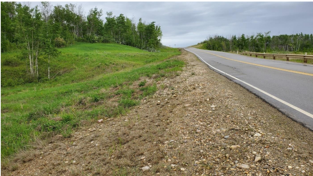
Photo 2 – Looking north at reconstructed sideslope above culvert inlet.
