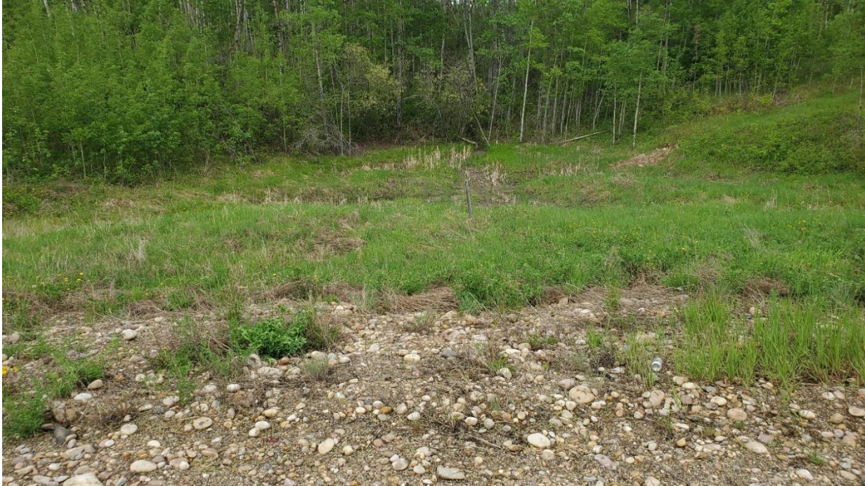
Photo 3: Looking northwest at new culvert inlet.
