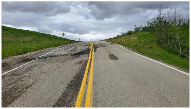
Photo 5, Site 15 – Looking north at diagonal crack intersecting the highway. There is a slight dip in the east lane on the south side (downslope) of the crack.
