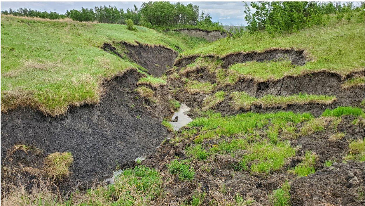
Photo 4, Site 14 – Looking south at slumping along tributary channel.
