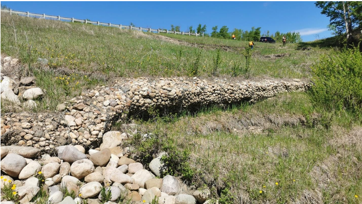
Photo 6 – Looking north at scarps above and below the gabion wall at the riprap apron.
