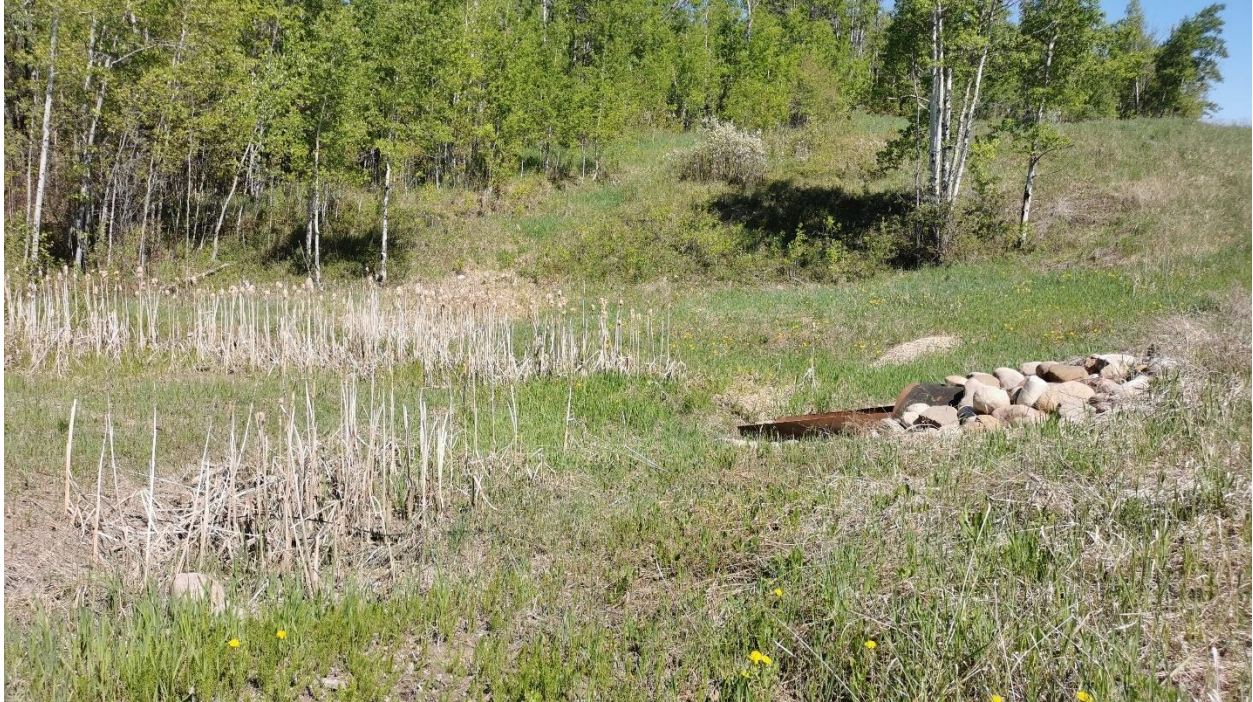
Photo 3: Looking north at new culvert inlet.
