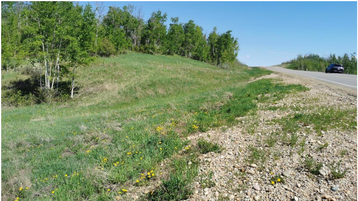
Photo 2 – Looking north at sideslope above culvert inlet.
