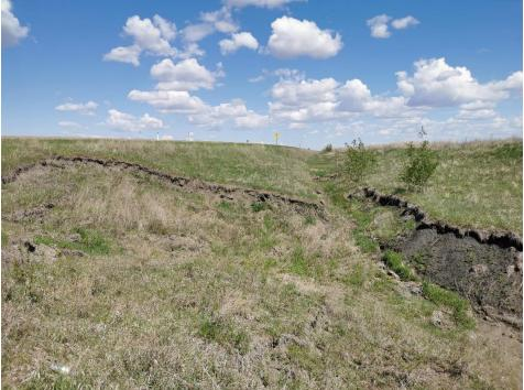
Photo 1, Site 14 – Looking north along the east ditch at increasing depth of erosion along the tributary.
