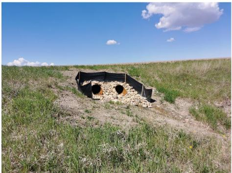
Photo 3, Site 14 – Looking at outlets of new SWSP twin culverts outlets which replaced older CSP culverts.
