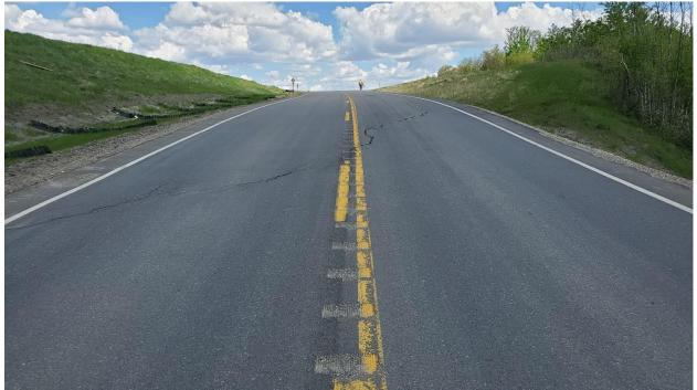
Photo 5, Site 15 – Looking north at diagonal crack intersecting the highway. There is a slight dip in the east lane on the south side (downslope) of the crack.
