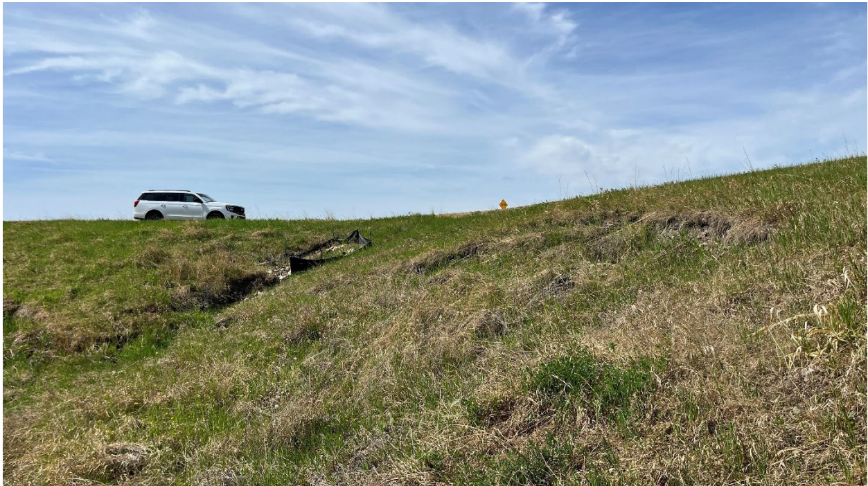
Photo 1, Site 14 – Looking southwest at slide scarp north of twin culverts that is retrogressing towards the highway.
