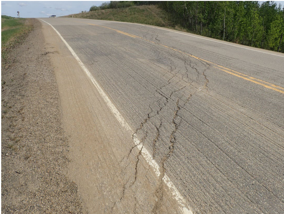
Photo 6, Site 15 – Looking northeast at the main crack. Scarp from road extends southwest into the treeline.
