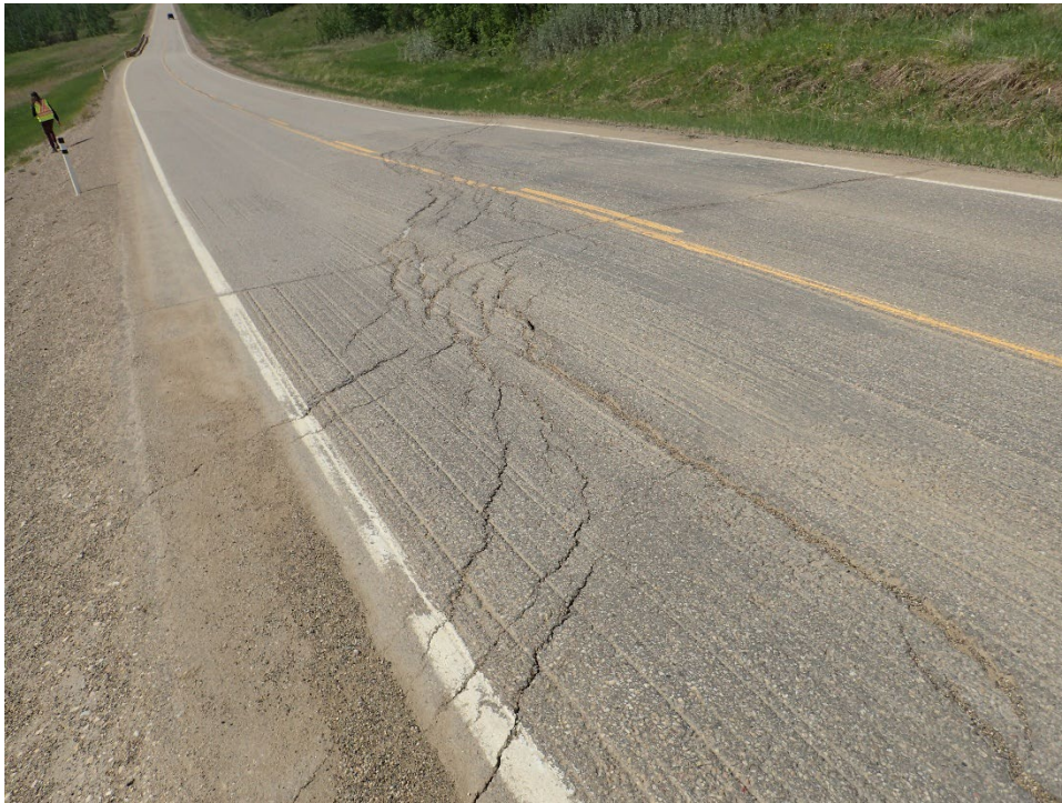
Photo 5, Site 15 – Looking southwest at diagonal crack intersecting the highway.
