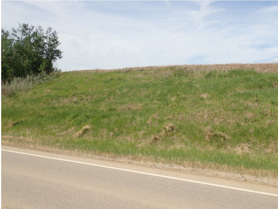
Photo 9, Site 15 – Looking southwest at backslope slump at valley crest.
