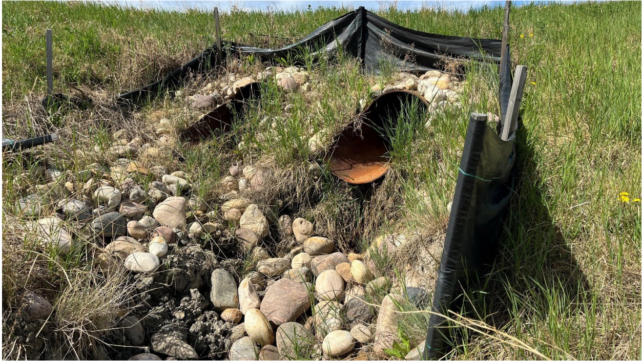
Photo 3, Site 14 – Looking at outlets of SWSP twin culverts outlets. The riprap apron at the north SWSP had collapsed.
