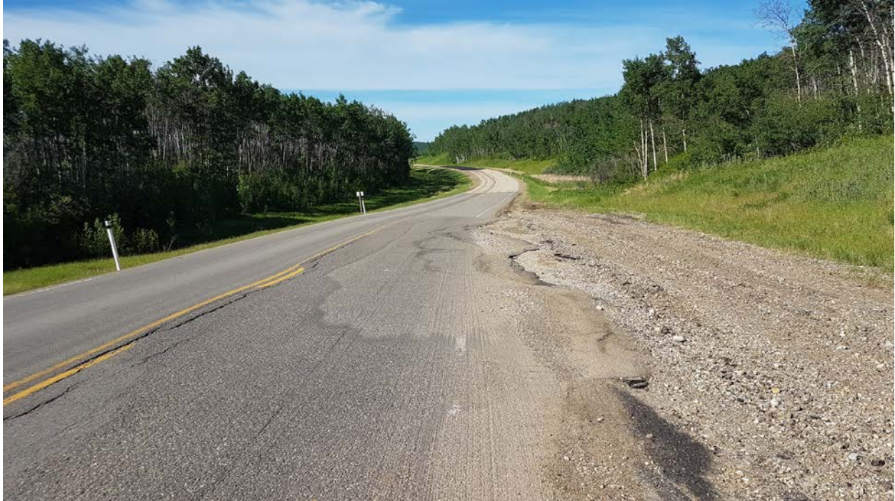
Photo 1 – Looking southwest at the southwest end of the main scarp crack through Site 11.
