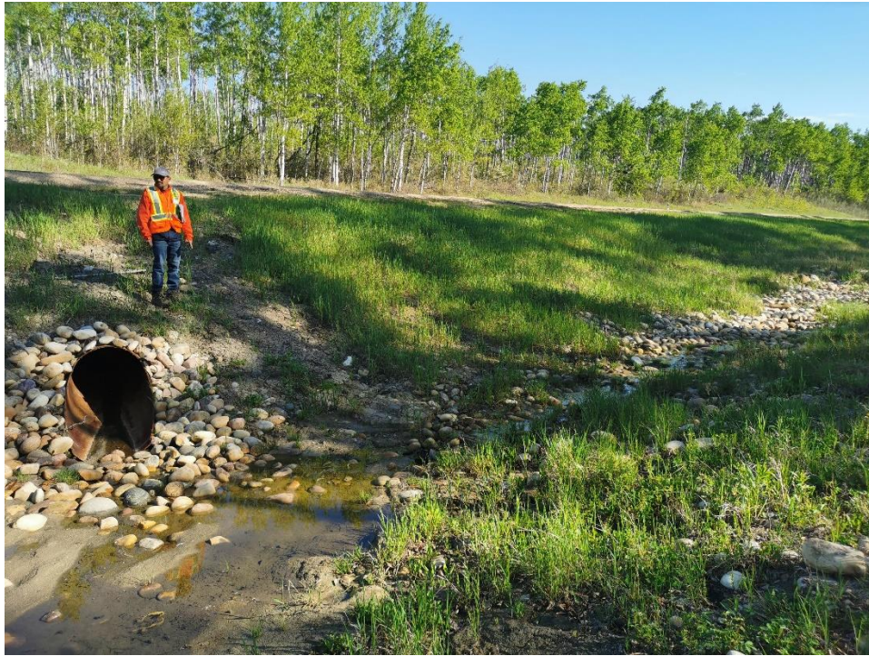
Photo 1 – Looking northeast along downslope ditch.
