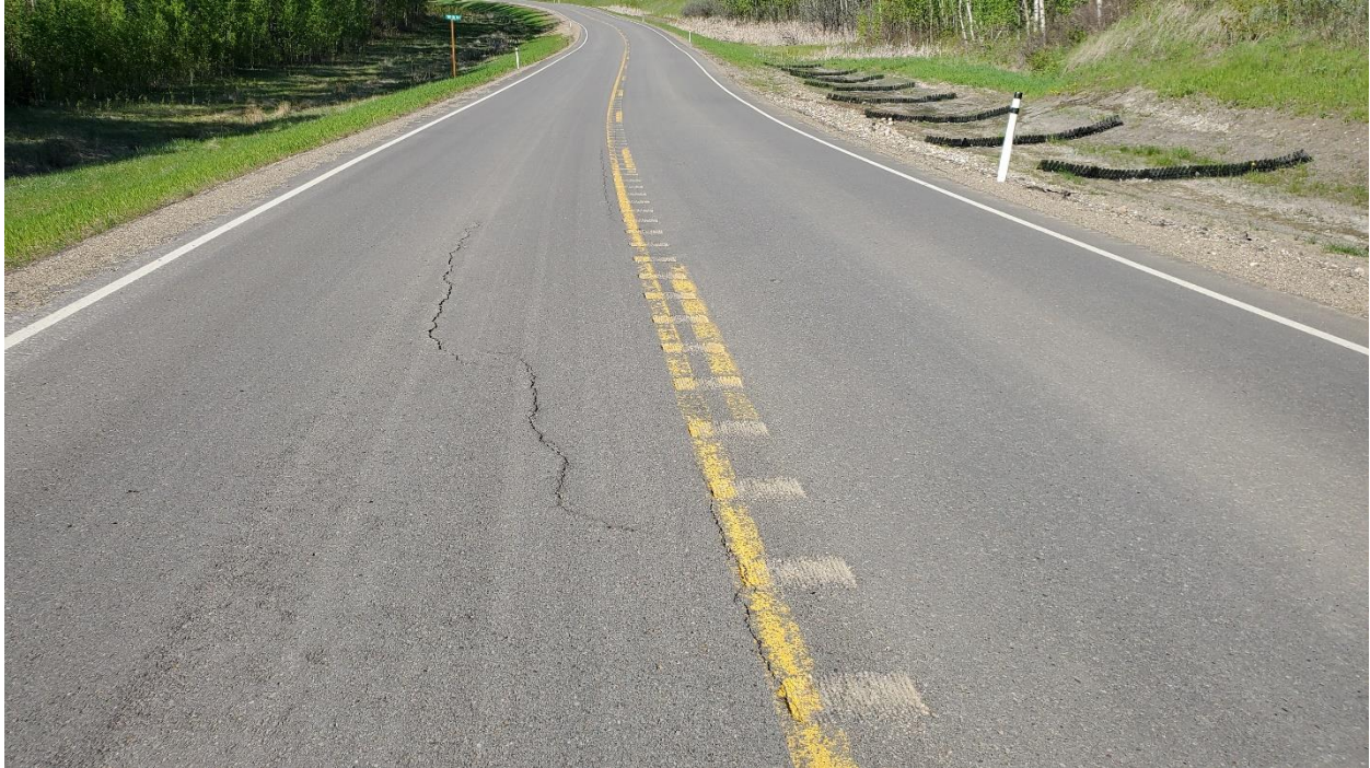
Photo 1 – Looking southwest at the southwest end of Site 11.
