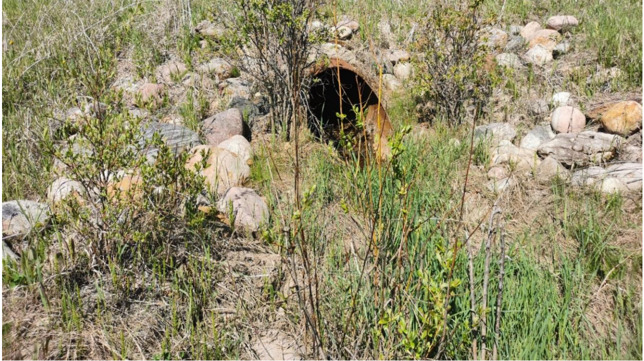
Photo 5, Site 12A – Looking at culvert liner outlet.
