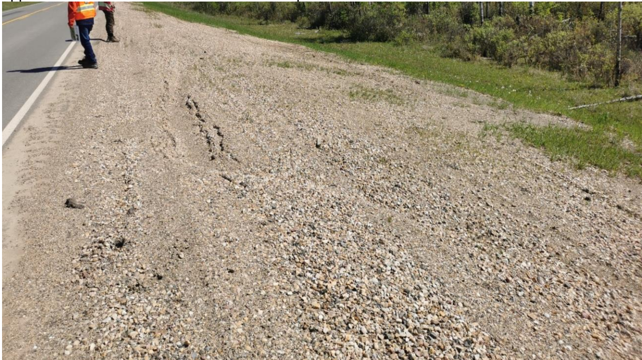
Photo 8, Site 12A – Looking north at top of gravel pile on downslope shoulder where a scarp is forming close to the highway.
