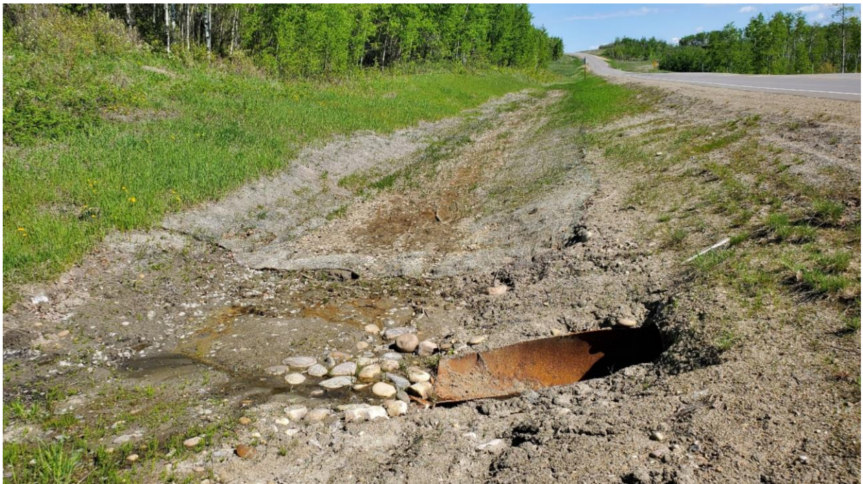
Photo 6, Site 12A – Regraded upslope ditch at culvert liner inlet.
