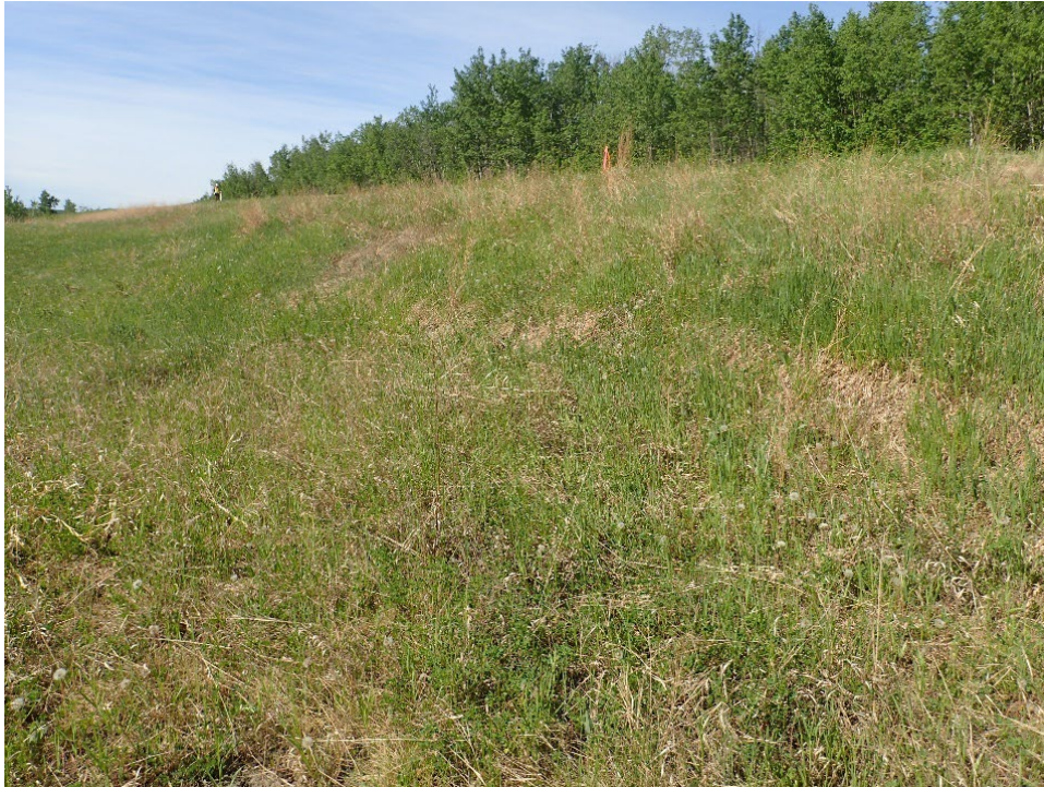
Photo 7, Site 12A – Looking south at toe roll downslope of where excess gravel appears to have been wasted on the sideslope. There appears to be some movement observed since the last inspection.
