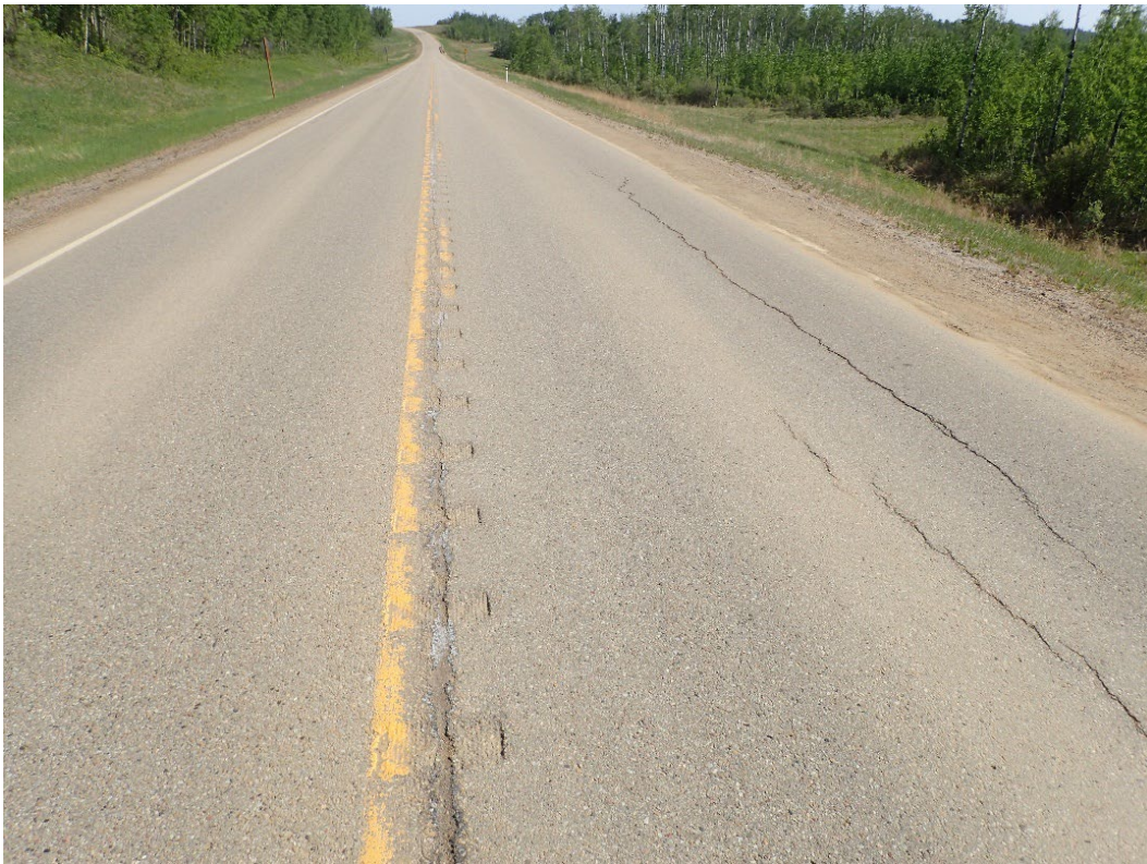
Photo 4, Site 12B: Looking north at cracks extending towards Site 12A.
