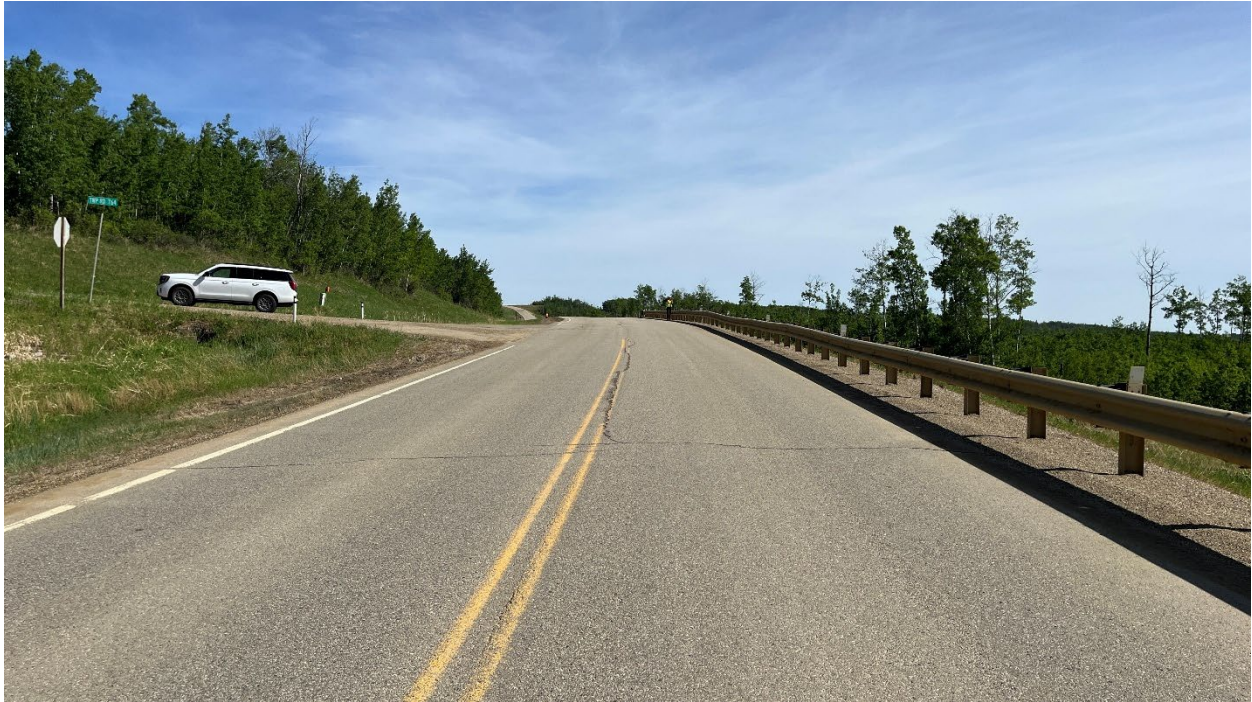
Photo 1, Site 12 – Looking northeast at the highway surface upslope of the toe berm location. There is a noticeable dip in the at the middle section of the guardrail.
