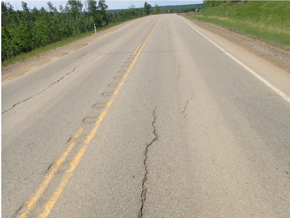
Photo 5, Site 12B – Looking south at cracks continuing to reflect through the 2021 overlay.
