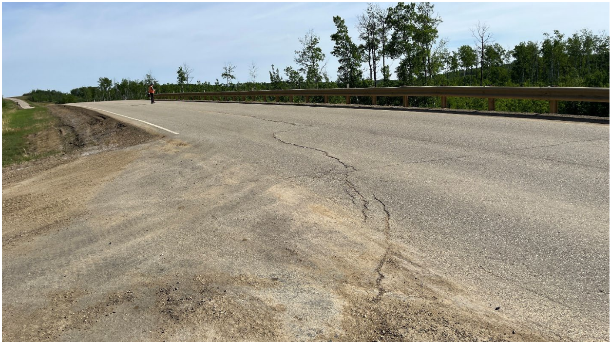
Photo 2, Site 12 – Looking northeast from the TR764 intersection at where the main scarp crack was located. The previous crack pattern is continuing to reflect through the 2021 overlay.
