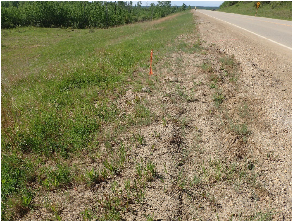
Photo 8, Site 12A – Looking south at the downslope shoulder, where a scarp had previously developed near the highway due to excess gravel placement.
