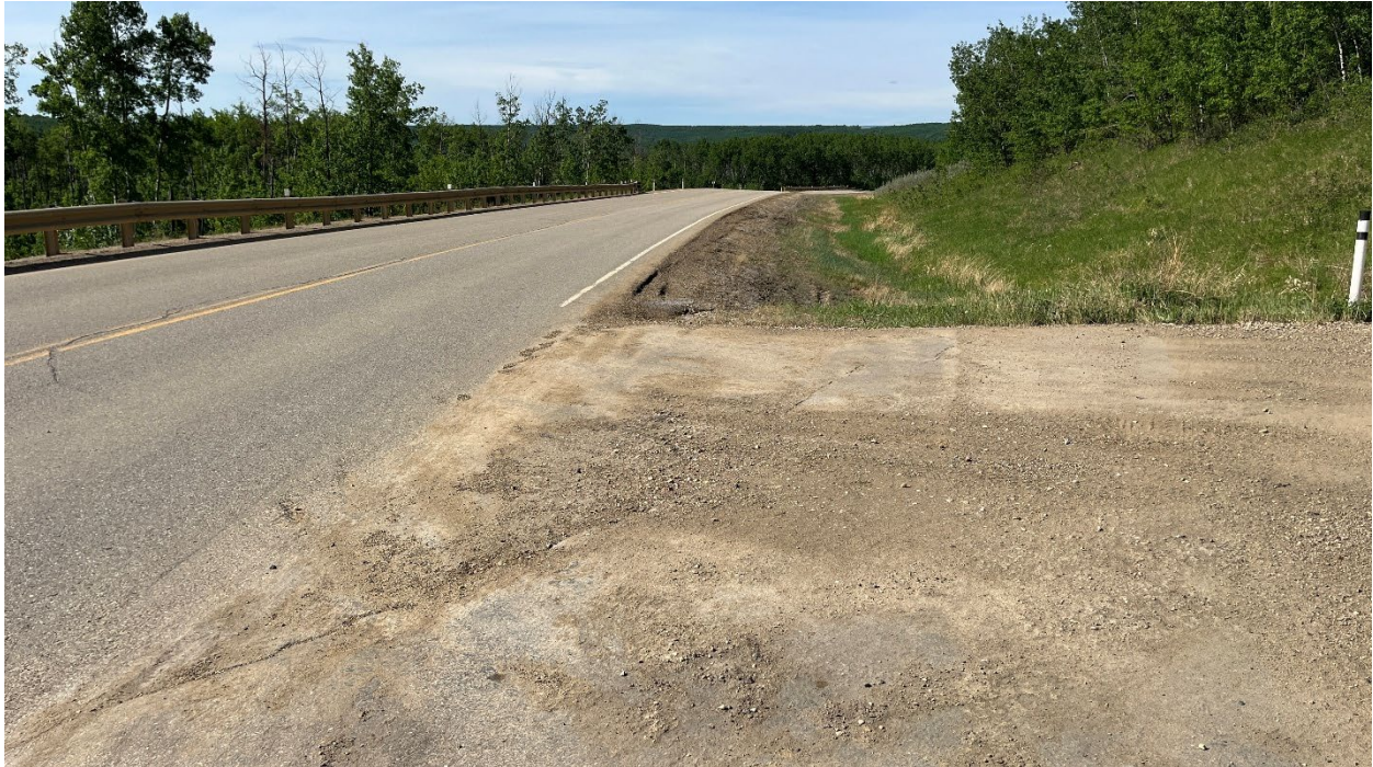
Photo 3, Site 12 – Looking southwest at the TR764 intersection where cracks have extended from the road surface towards the southwest ditch.
