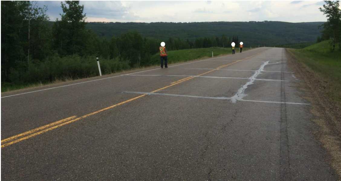
Photo 1 (looking north). No indications of pavement distress or deformation were observed.
