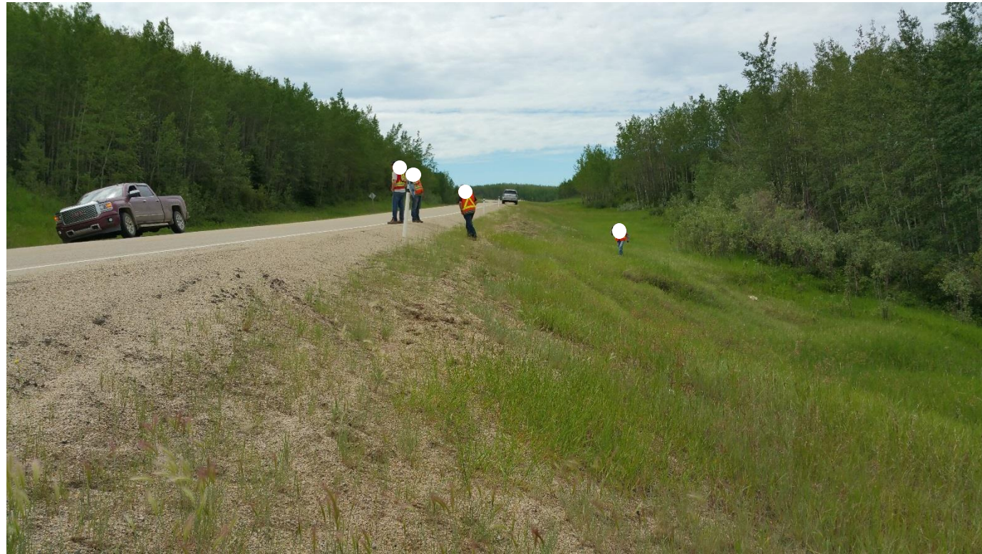
Photo 1: (looking south) No indications of pavement distress or deformation were observed.
