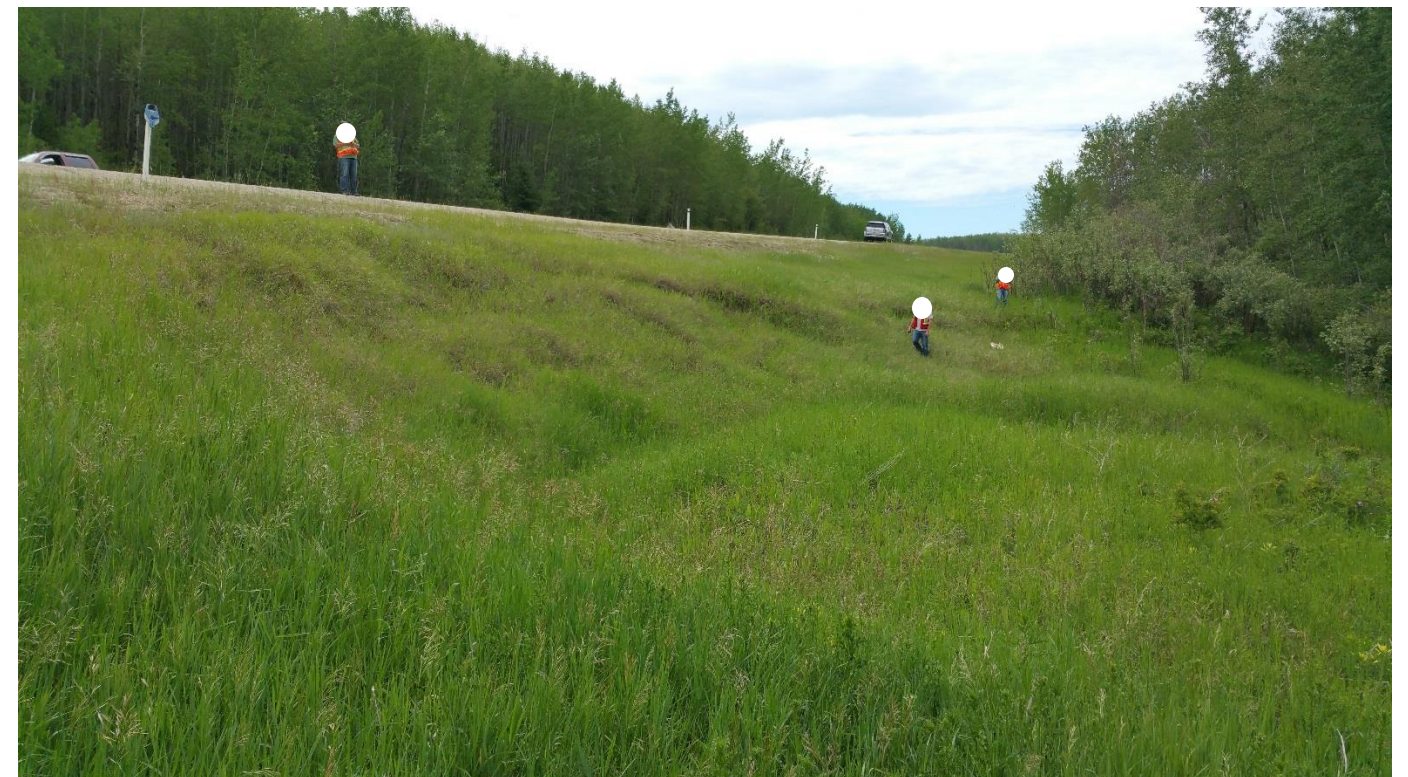
Photo 2: (looking south) Distance between the edge of the pavement and backscarp was unchanged from July 2014.
