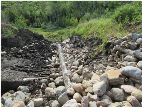
Photo 7. (Aug. 6/19) Looking east at the mudflow below the severed drainpipe at the sheet pile wall below former slide 2.
