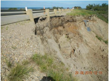
Photo 14 (Aug20/19) Taken by Erwin Kurz of TRANS, this photo shows indications of additional backscarp retrogression toward the highway (compare to Phot 3)
