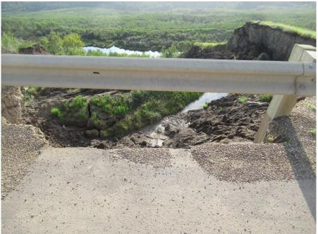
Photo 4. (Aug. 6/19) Looking east down the centre of the new landslide toward the Heart River valley.
