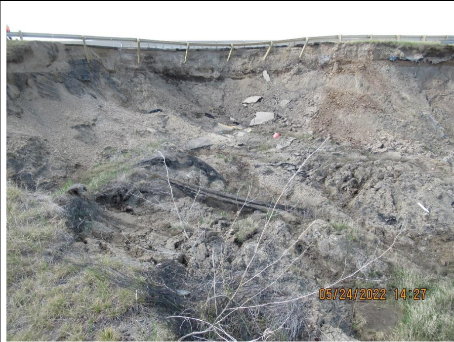
Photo 3. Looking upslope towards the west at the main scarp of Slide 1A from the lower south flank.
