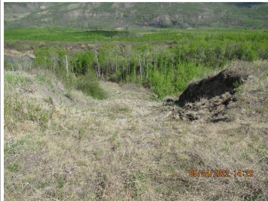
Photo 7. Looking east at mud flow at the location of former Slide 3, which has been more active since 2021. Decreased vegetation since previous inspection indicative of active soil movement.
