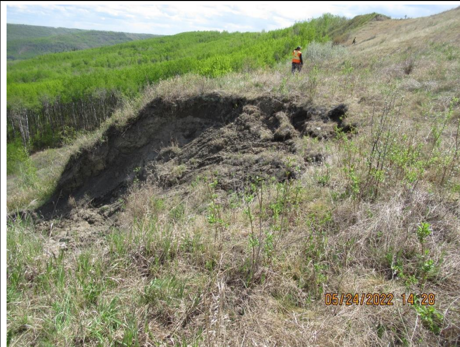
Photo 5. Looking south at the slide south of the sheet pile wall with recent retrogression visible.
