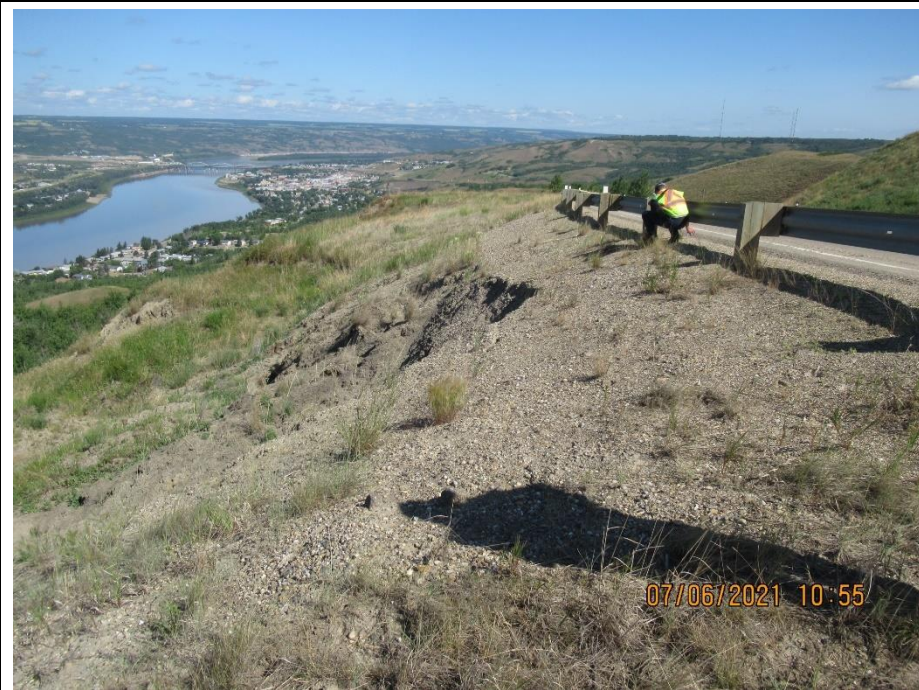
Photo 5. Looking north from downslope of the SBL of Hwy 744:04 at km 57.63. Increased dropdown within the disturbed slide mass. Headscarp has expanded to the previously observed tension crack location with 0.7 m of additional retrogression since 2020, offset from the guardrail is now at 2.5 m.
