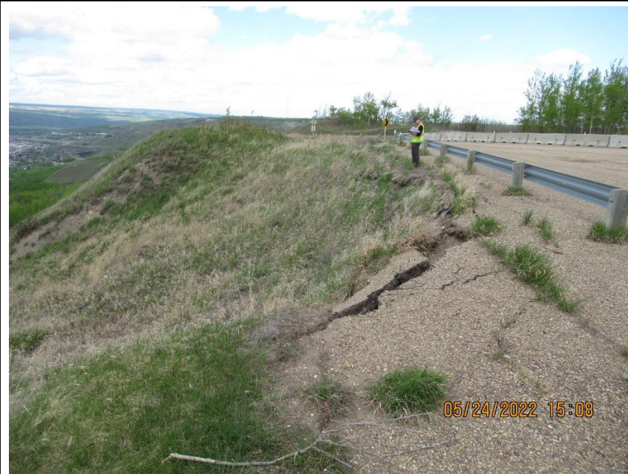
Photo 2. Looking northeast along backscarp of Slide 2 which is 0.6 m from the parking lot guardrail. Some localized main scarp retrogression, flank retrogression and additional pavement cracking since 2021.
