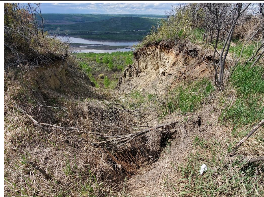
Photo 8. Looking at the top an erosion gully located at the southern edge of the site, approximately 50 m south of the Slide 4 area. Gully is offset approximately 70 m west of the highway.
