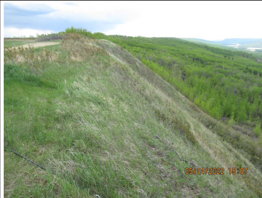
Photo 1. Looking southwest from above Slide 2 towards Slide 4 (No change since 2021).
