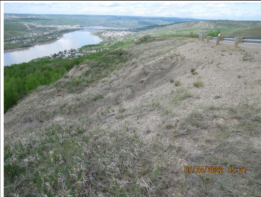
Photo 5. Looking north from downslope of the SBL of Hwy 744:04 at km 57.63. Increased dropdown within the disturbed slide mass. Headscarp has retrogressed 0.5 m since 2021; offset from the guardrail is now at 2.0 m.
