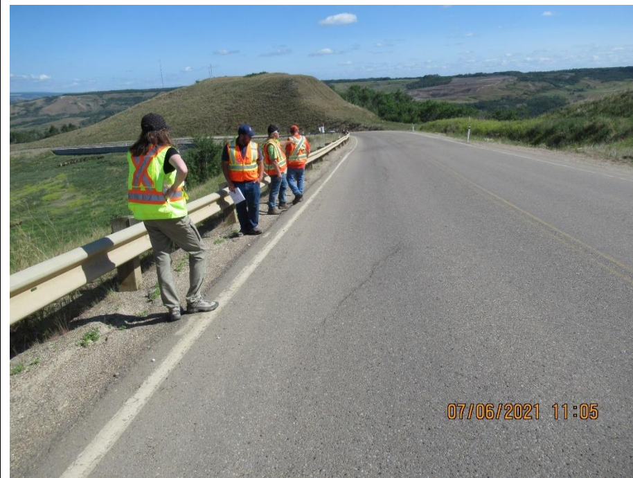
Photo 1. Looking northeast along the centerline of Hwy 744:04 at km 57.75 at the north end of the 2014-2015 realignment. No major changes observed from the 2020 pavement condition apart from some increased localized settlement at the shoulder.
