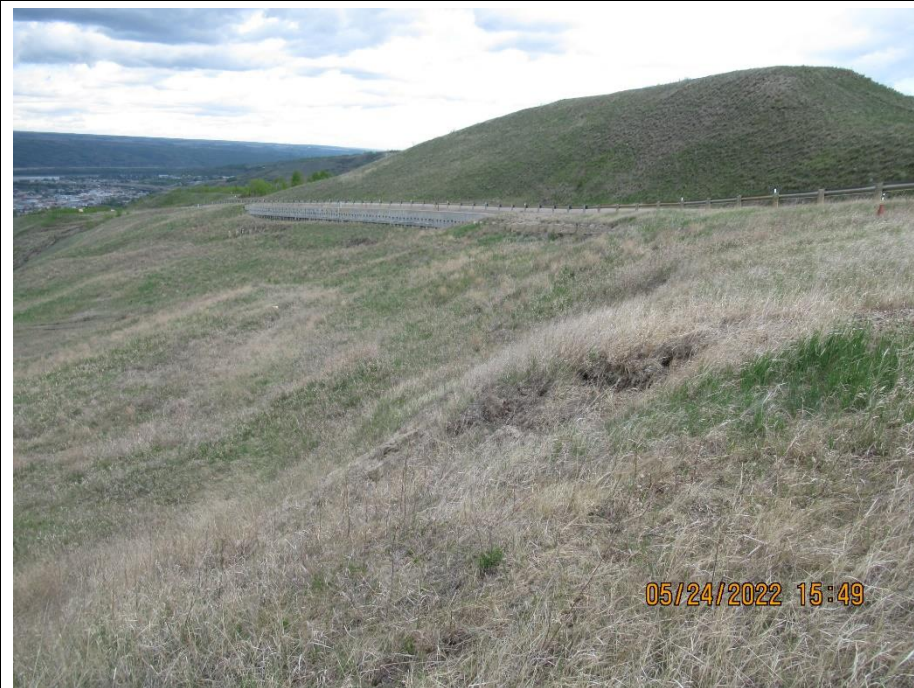
Photo 2. Looking north along the west sideslope of Hwy 744:04 at km 57.94 below the old pile wall.
