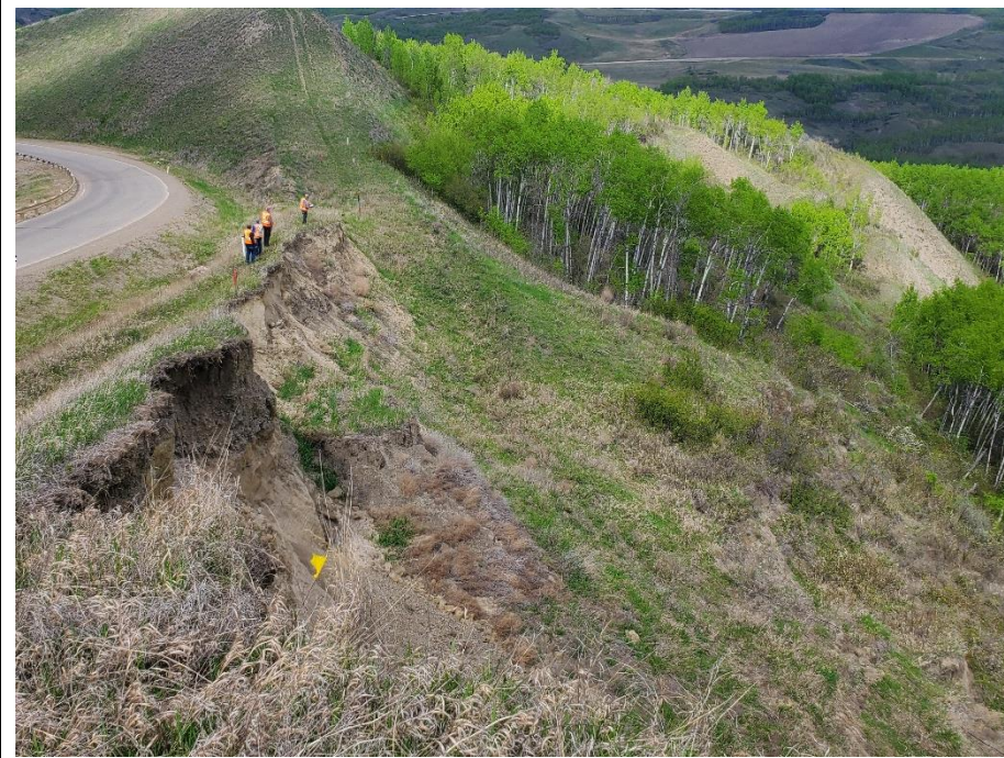
Photo 3. Looking northeast along the backscarp of the landslide at the top of the Heart River valley on Hwy 744:04 at km 57.8. No change to the location of the main scarp. More erosion and downslope movement within the upper scarp face.
