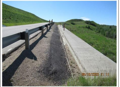
Photo 11. Looking south along the top of the "Makeout" pile wall. ACP shoulder protective cover was in good condition. Previous ridge of sediment building beneath the guardrail was removed/washed away. Drainage trough was relatively clear and functioning.
