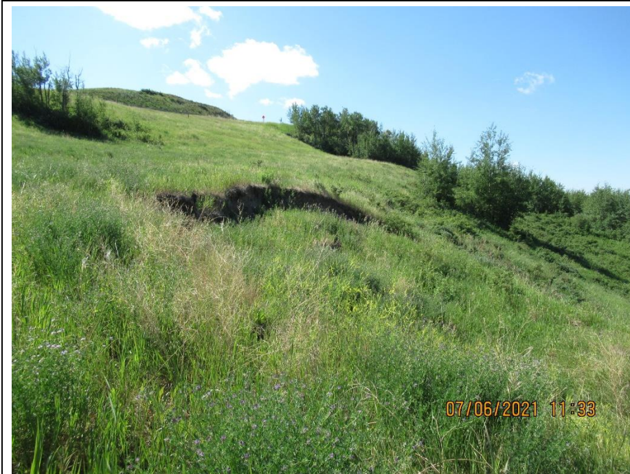
Photo 3. Looking south at a scarp in the bench below the south end of the wall with approximately 1.5 m maximum drop. Area is well vegetated with no significant expansion or downslope movement since 2020.
