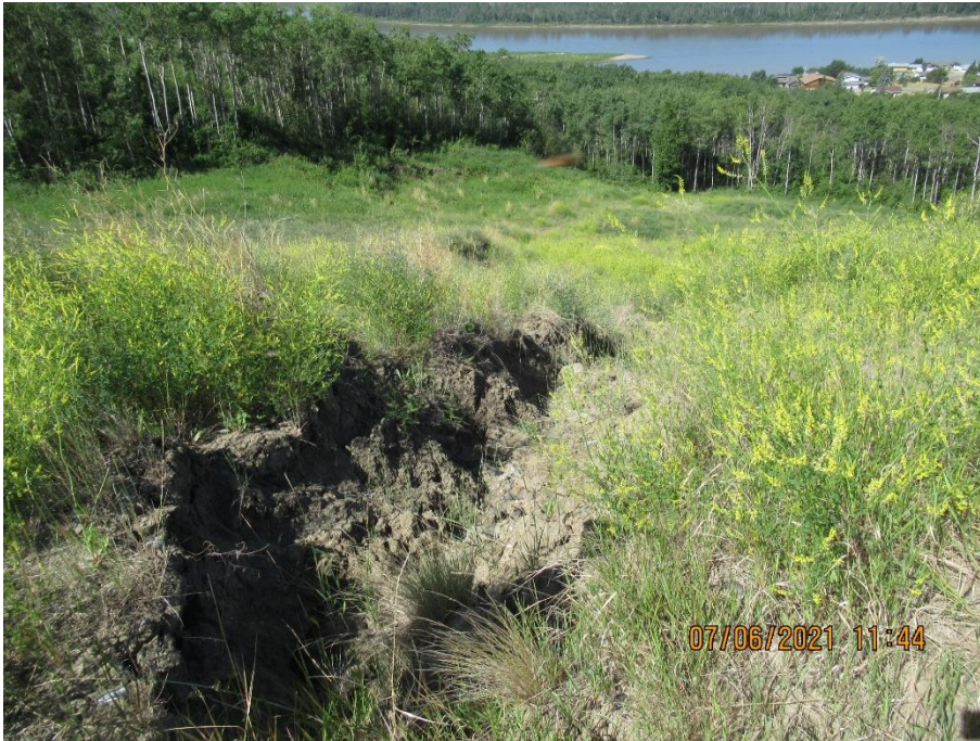
Photo 5. View downslope towards the head of an active erosion gully approximately 40 m downslope from the north end of the pile wall and disconnected drainpipe further upslope.
