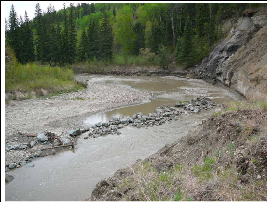
Photo 13. The Heart River is now flowing entirely on the west side of the channel, having bypassed the rip rap. Erosion is occurring along the toe of the slope, removing debris (foreground) and undercutting the rock slope.
