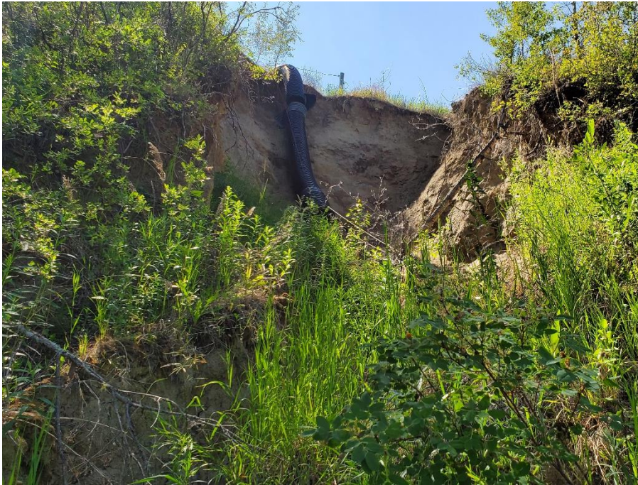
Photo 5. Looking southwest from below the scour caused by the breakage in the CNR CPP Trunk pipe. There has been some retrogression and lateral expansion at the gully headwall since 2020.
