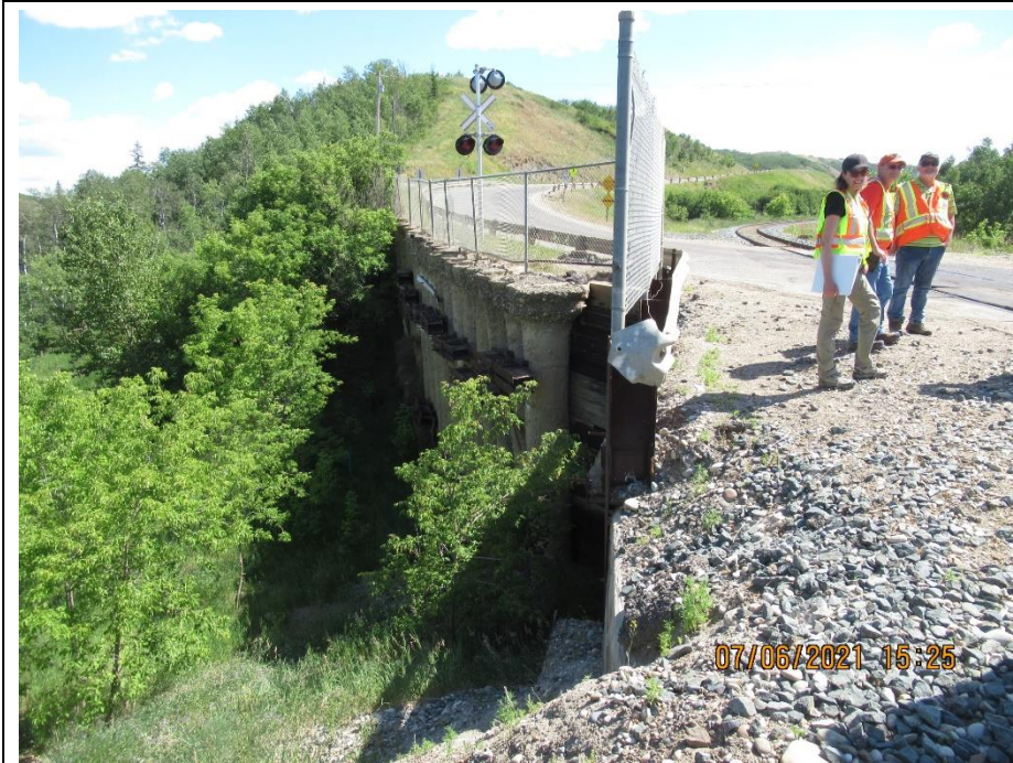
Photo 1. Looking southeast from the north end of the CNR pile wall. Apart from ongoing ravelling and cement spalling between the piles there was no significant change observed at the downslope face of the pile wall or slope directly below since 2020.
