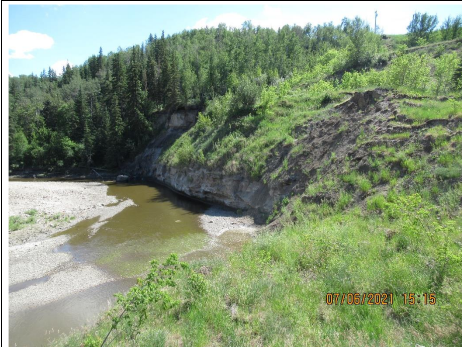
Photo 7. Looking east along the toe of the lower landslide. Lower slide activity and toe erosion at the riverbank is active.
