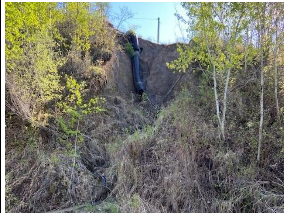
Photo 5. Looking southwest from below the scour caused by the breakage in the CNR CPP Trunk pipe. There has been some retrogression and lateral expansion at the gully headwall since 2021.
