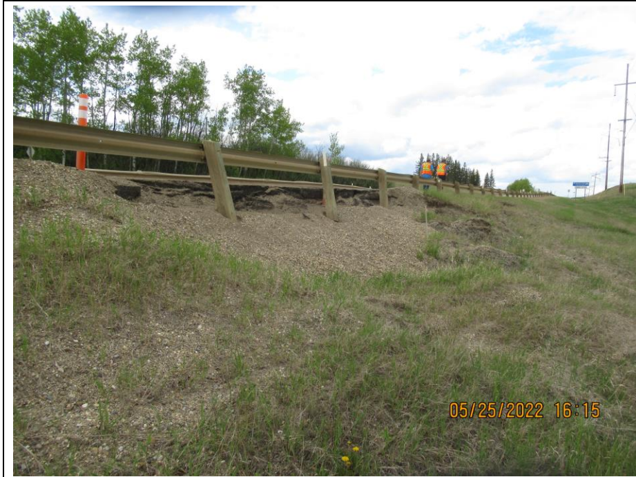
Photo 65-2. Looking north along the east side of the highway embankment towards an active main slide scarp (45+015) first identified in 2016. Slightly increased retrogression since 2021, minor change to the scarp height.
