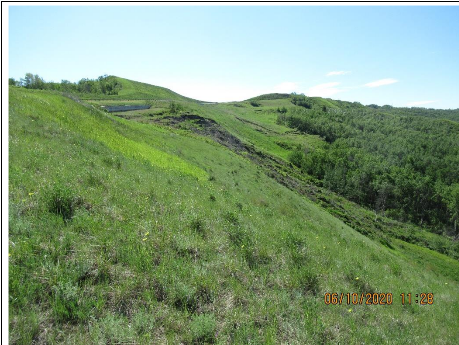
Photo 5. Looking southeast at the lower slide area below the wall. Very active in lower slope.
