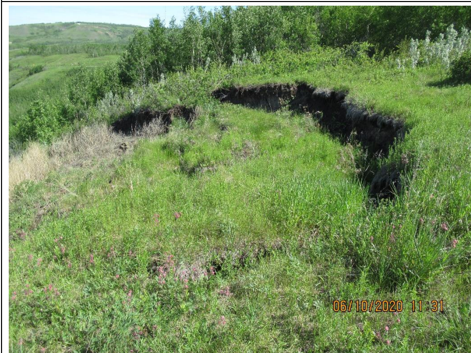
Photo 6. New slide area (first observed in 2019) approximately 100 m NW of the north end of the pile wall. No major change at the headscarp since the 2019 inspection. More movement downslope was noted.
