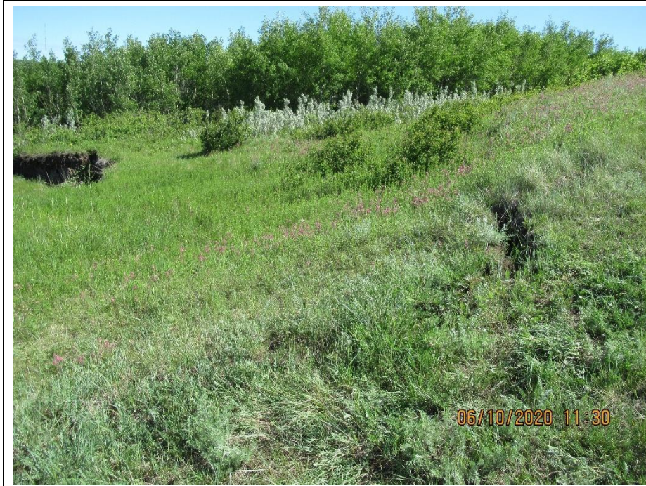
Photo 7. Same location as Photo 6 looking northeast at one of three tension cracks observed upslope from the slide scarp. Tension crack had a minimum offset of approximately 50 m from the highway, no change from the 2019 condition.
