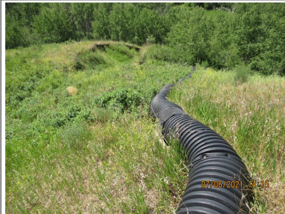
Photo 4. Looking southwest at km 58.9 at CPP drain and erosion gully further downslope. Gully is well vegetated and has not visibly changed from 2020.
