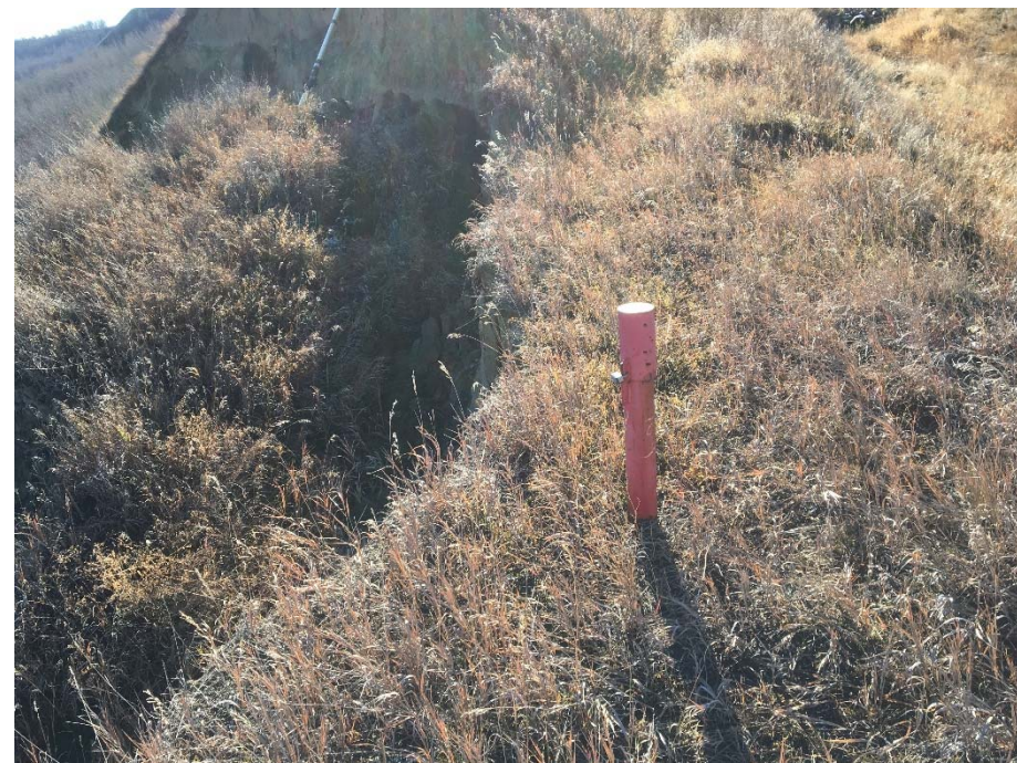
Photo 5. Looking south at the south flank of the Heart River side slide from the former ATCO pipeline right-of-way. The scarp is 0.4m from SI10-04 and the drop along the scarp is at 4.5 m.
