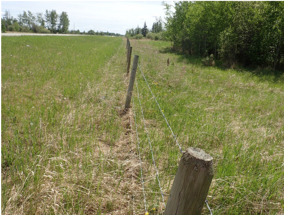
Photo 3: Looking south along west ditch at portion of fence that is tilting.
