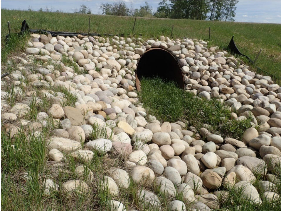
Photo 7: Looking southeast at SWSP culvert outlet.
