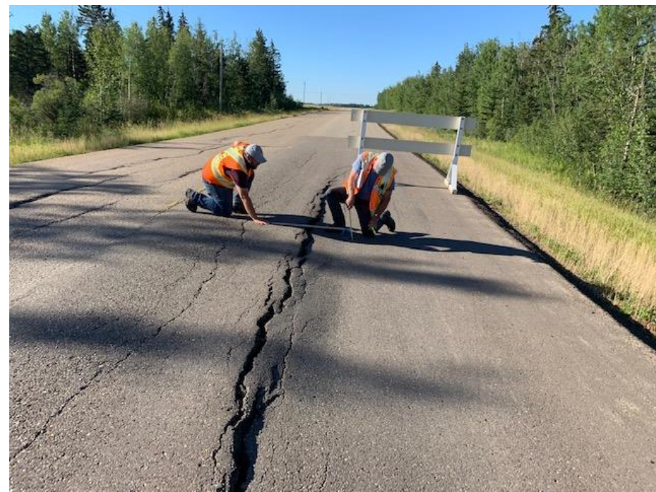
Photo 3. Looking south at scarp drop being measured.
