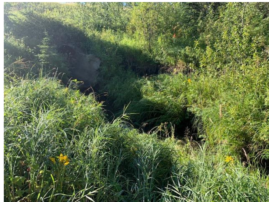
Photo 7. Looking east at 1.8 m diameter corrugated multi- plate.
