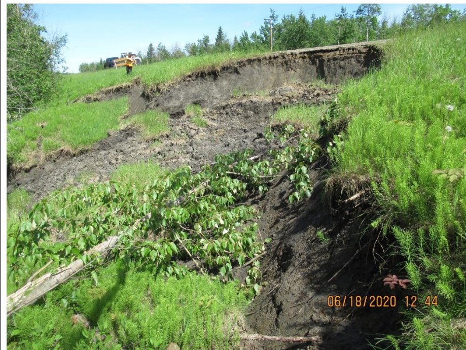
Photo 3. Looking northeast towards backscarp and slabs of soil that have fallen downslope.
