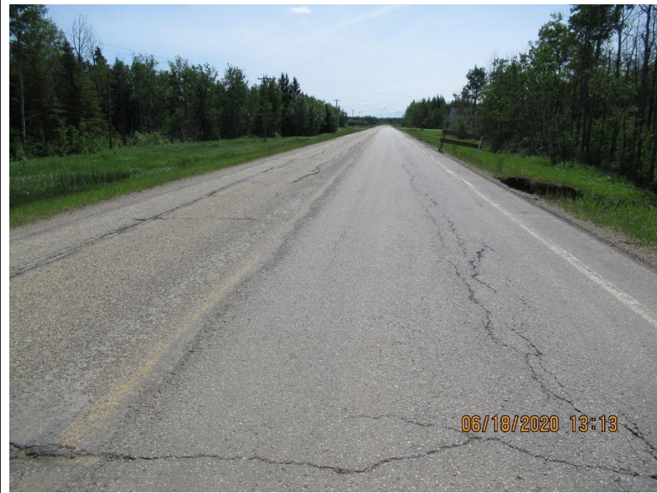
Photo 10. Looking south at highway 749.
