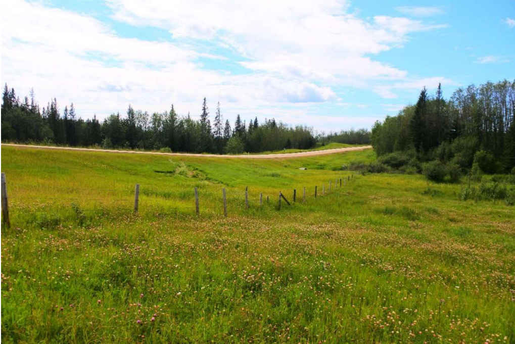
Photo 9 – Looking south at where linear disturbance along toe berm which might be a scarp or previous equipment rutting/disturbance; however, was grown over in July.
