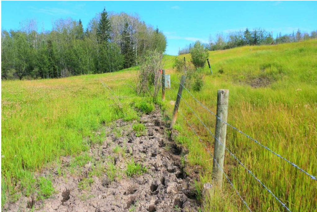
Photo 7 – Looking north at where soil was wet and had rutting from livestock.
