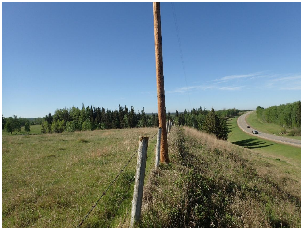
Photo 2 – Looking south at tilted power pole on east backslope.
