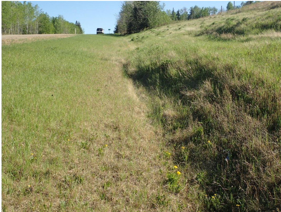
Photo 8 – Looking north at toe roll of backslope slumps.
