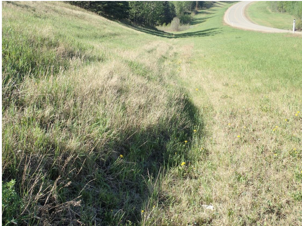
Photo 9 – Looking south at toe roll of backslope slumps.
