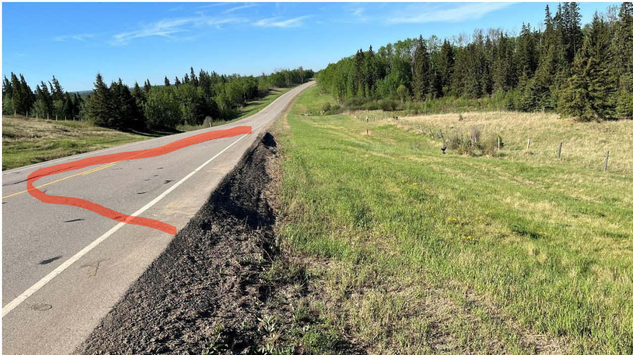
Photo 11 – Looking south at main crack (highlighted in red) near the north end of the site.
