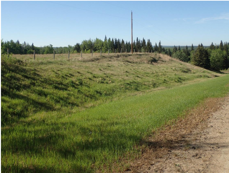
Photo 1 – Looking southeast at east backslope slumps.
